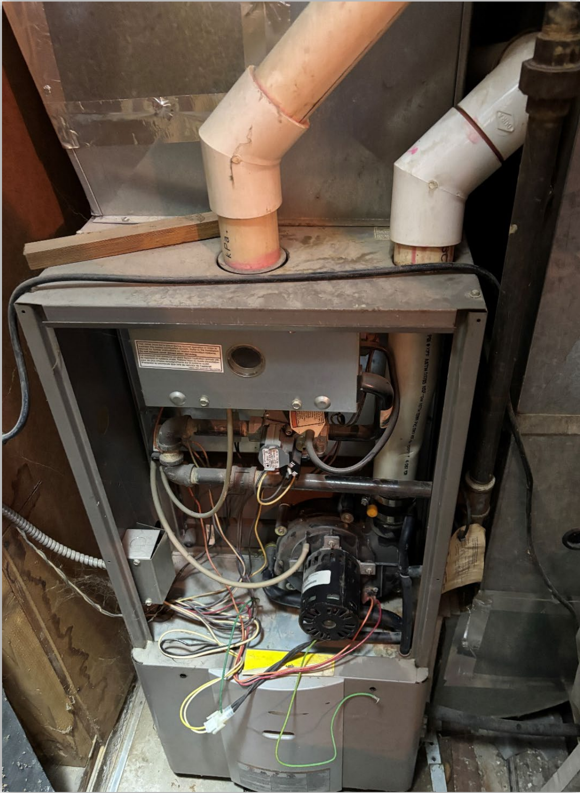
Image 3 – Gas furnace with upper cover removed as found after incident.
