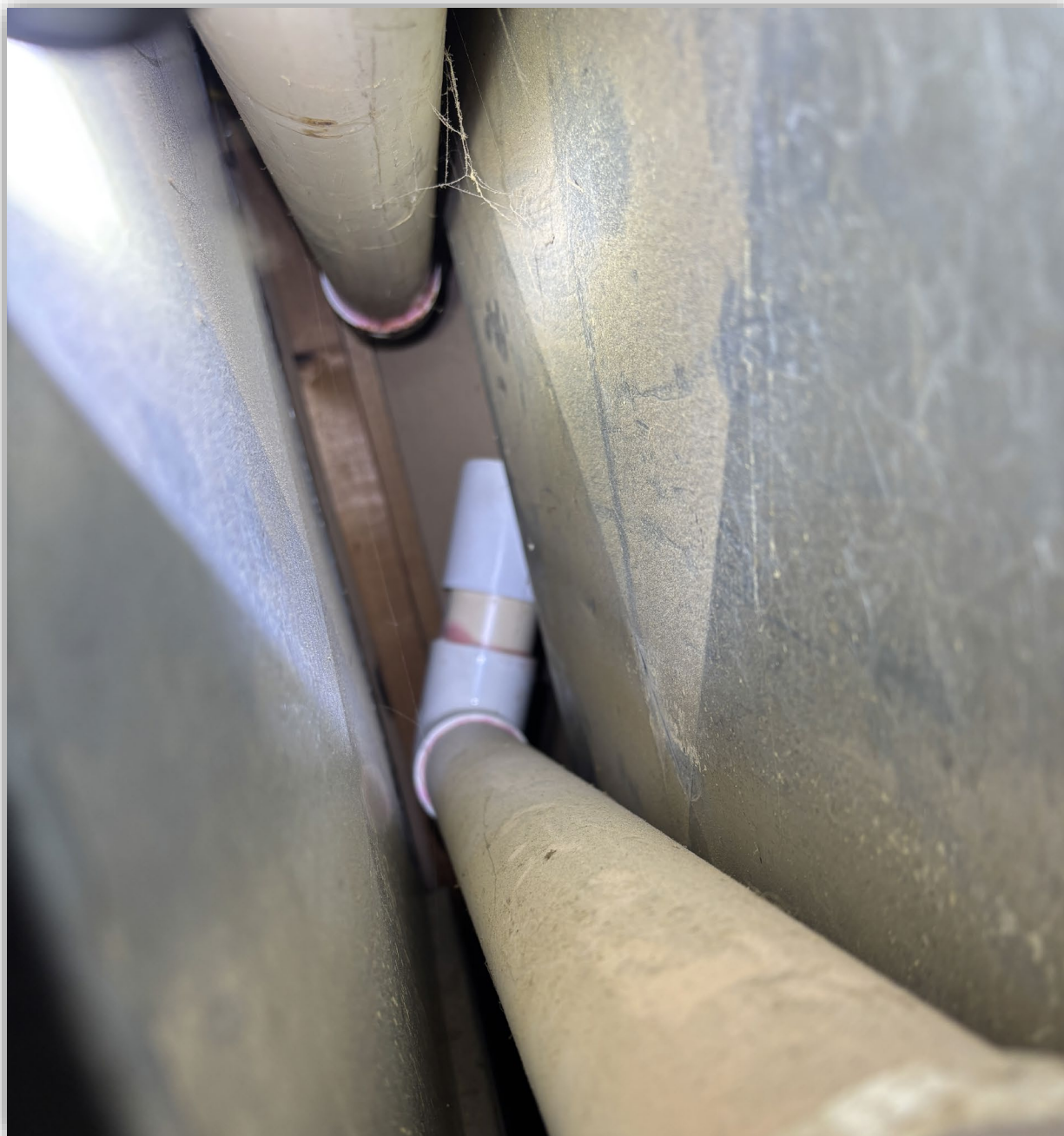
Image 6 – Disconnected flue vent pipe behind furnace as found after incident.
