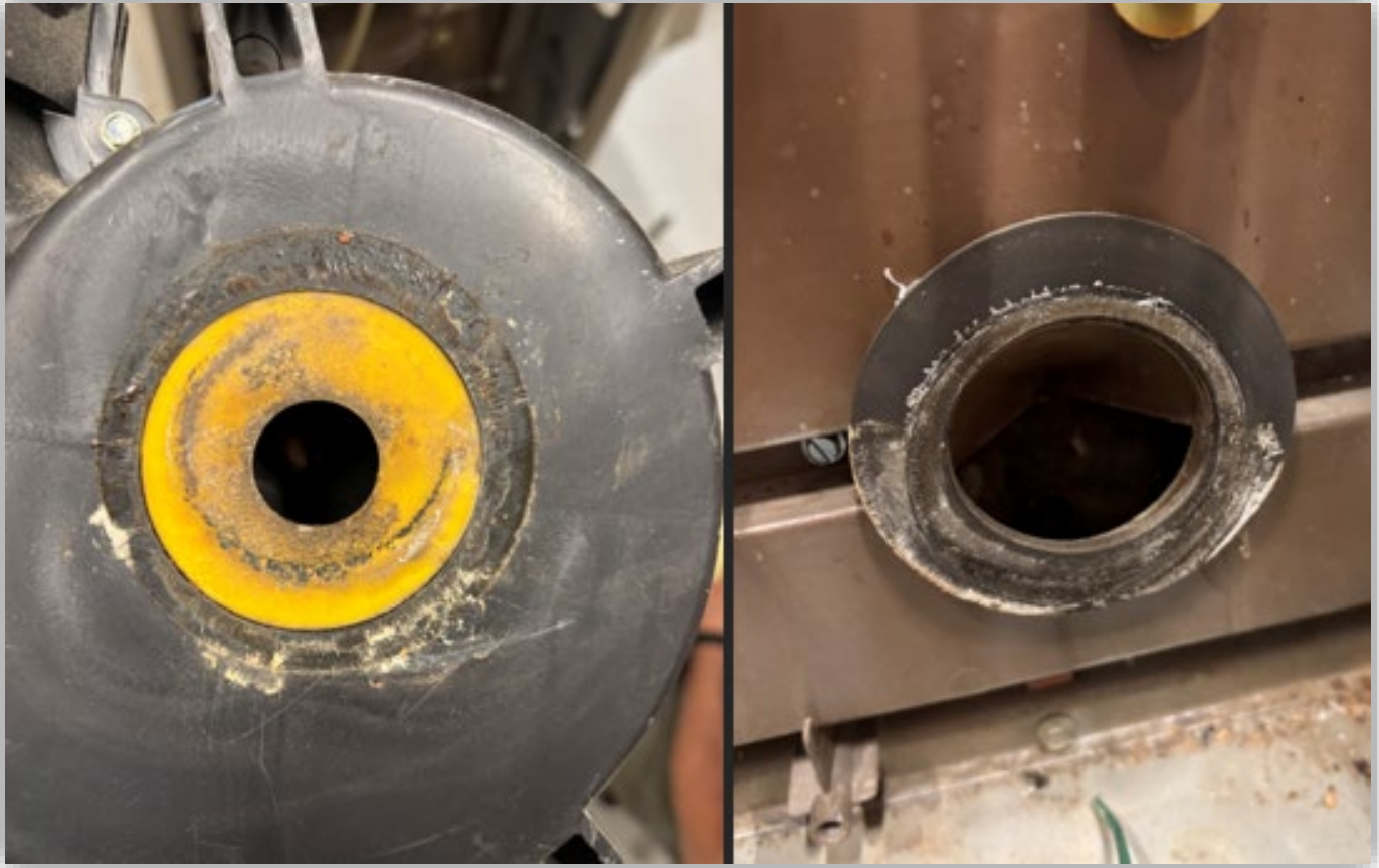
Image 5 – Draft inducer motor connection to furnace showing condensate leakage from improper seal from loose connection.
