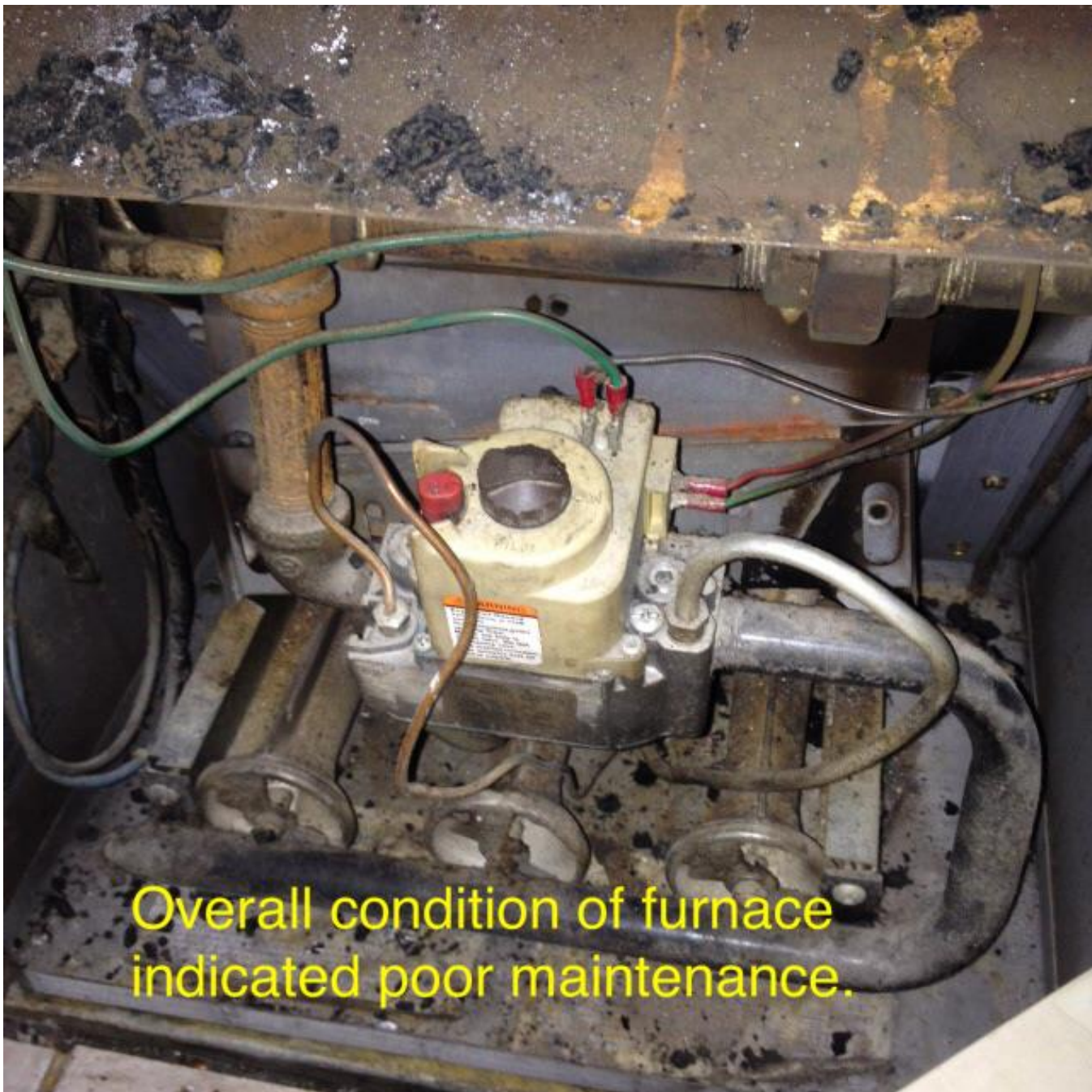
Image 1 – Dirt, debris and carbon deposits indicate extended furnace operation without service and maintenance. The last indication of furnace service by a qualified individual was six years prior.
