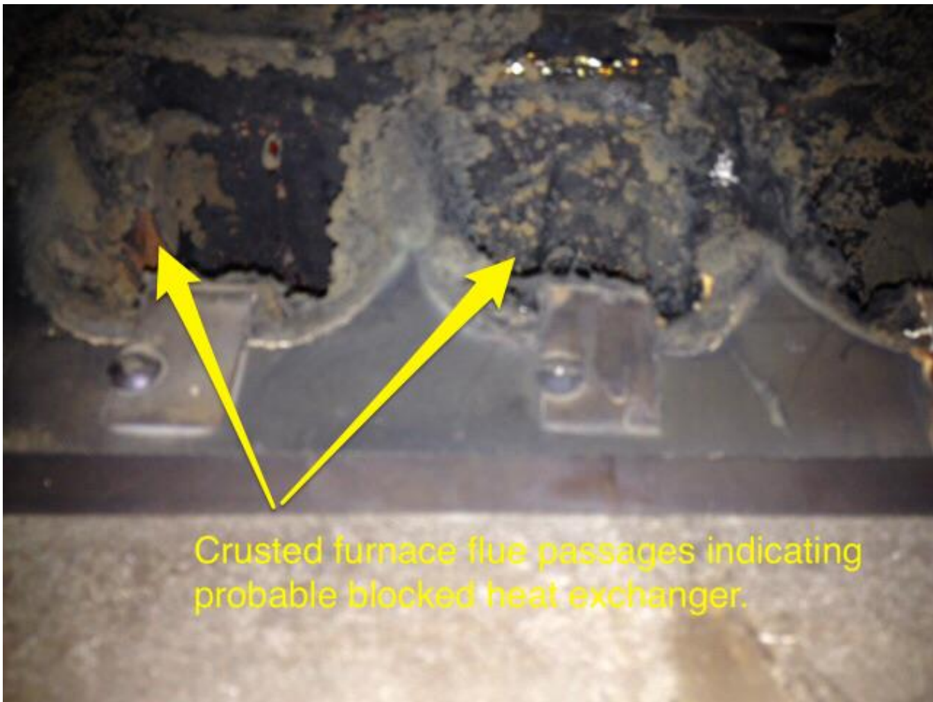
Image 4 – Deposits found at the outlets of the heat exchanger passages indicate incomplete combustion and the possibility of restricted or plugged flue passages that can allow the flue gas containing carbon monoxide to spill into the home.
