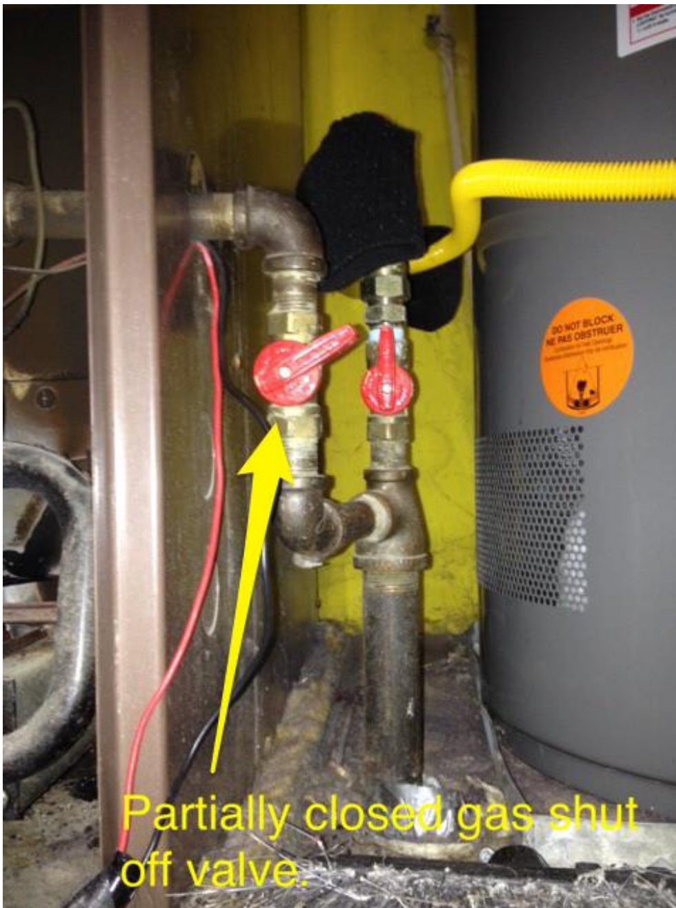
Image 3 – A partially closed valve can restrict the amount of gas required by the furnace and lead to incomplete combustion and the production of elevated levels of carbon monoxide.
