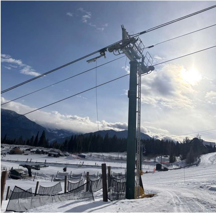
Image 4 – The remaining portion of the hanger arm lodged in the sheaves of tower 1, resulting in the need for a manual evacuation.
