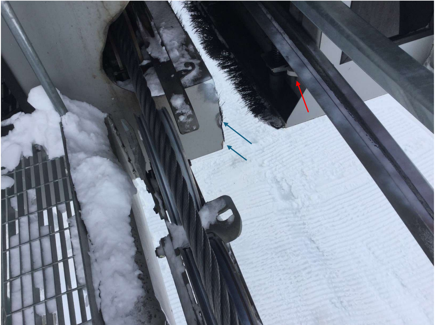
Image 11 – Photograph taken by a Safety Officer in 2017 showing the missing rubber bumper dampers on the guide rails (red arrow). Impact marks to the station rail can also be seen (blue arrows).
