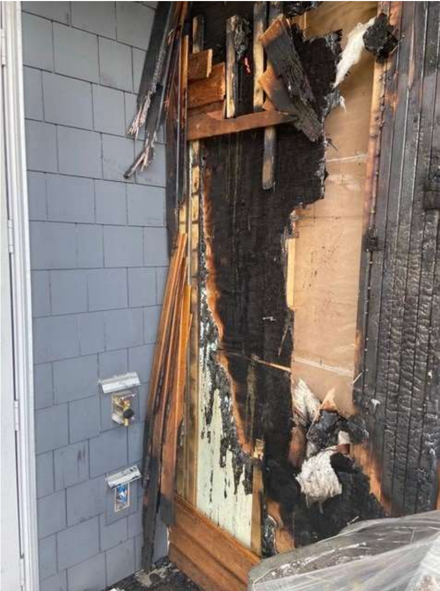
Image 1 - Damage to party wall where the portable BBQ was being operated
