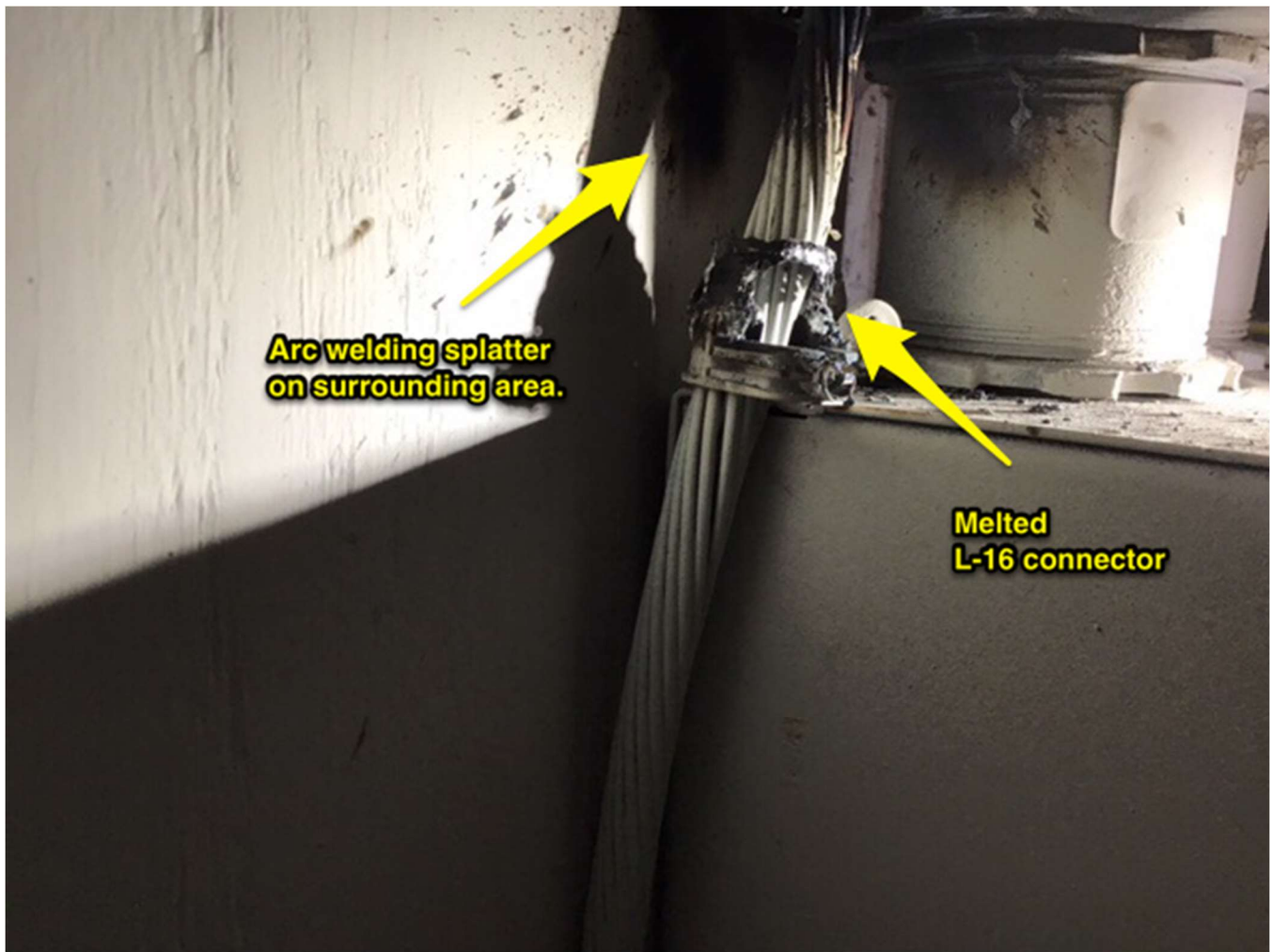
Figure 3 – Close up of metal connector melted
