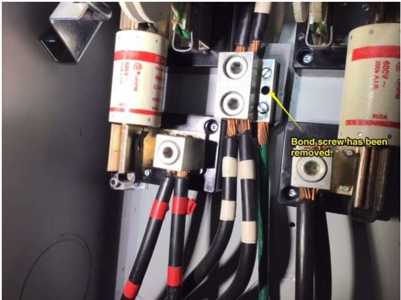
Figure 1 - Service disconnect switch with the required system bonding jumper screw missing
