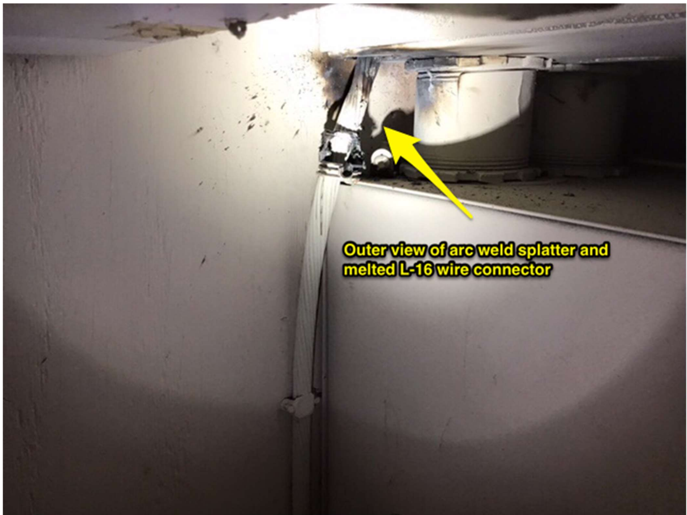
Figure 2 – Connector melted from passing current to the neutral conductor
