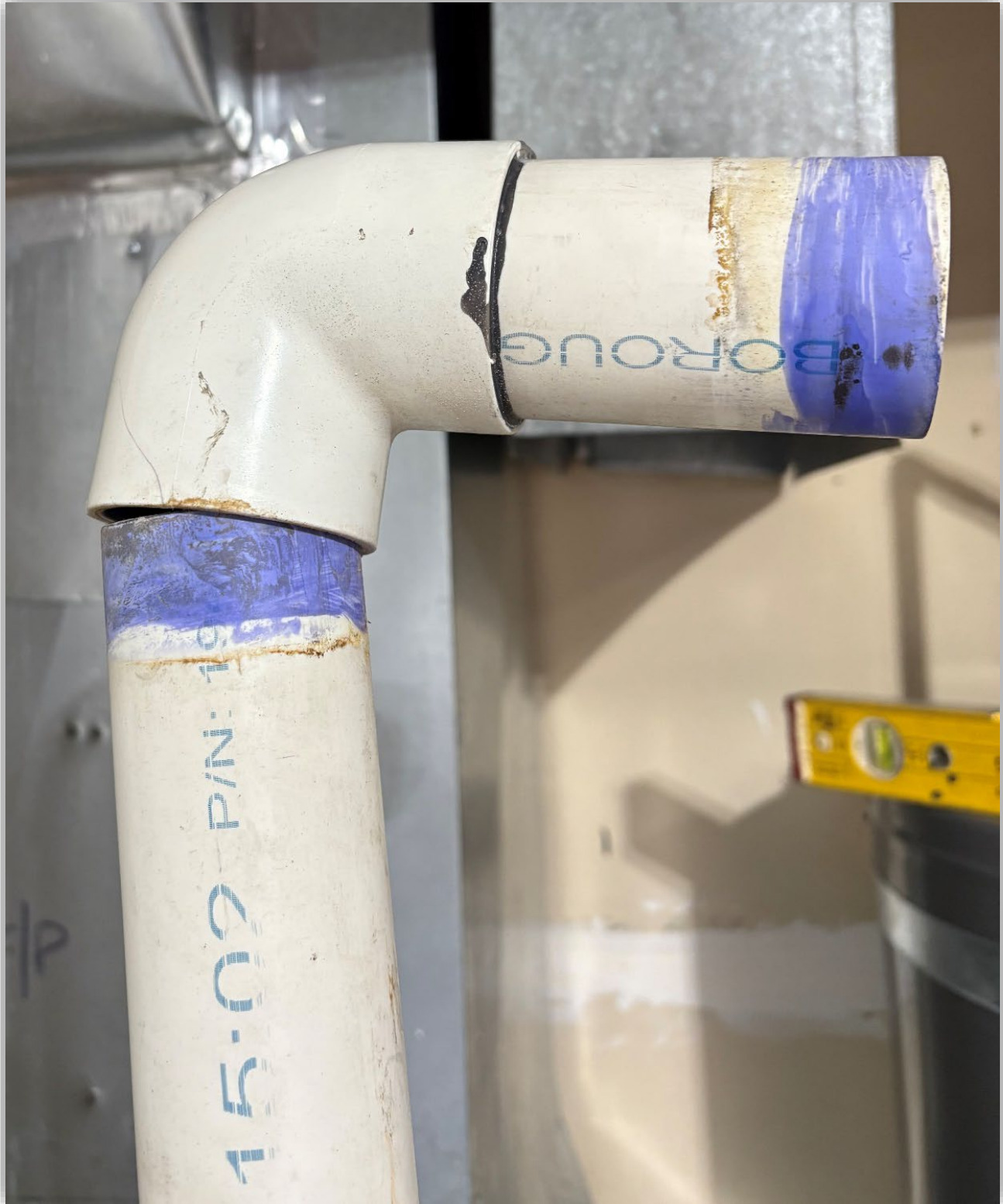
Image 4 – Venting joints originally installed with primer only and without glue. Both joints were able to be pulled apart by hand.
