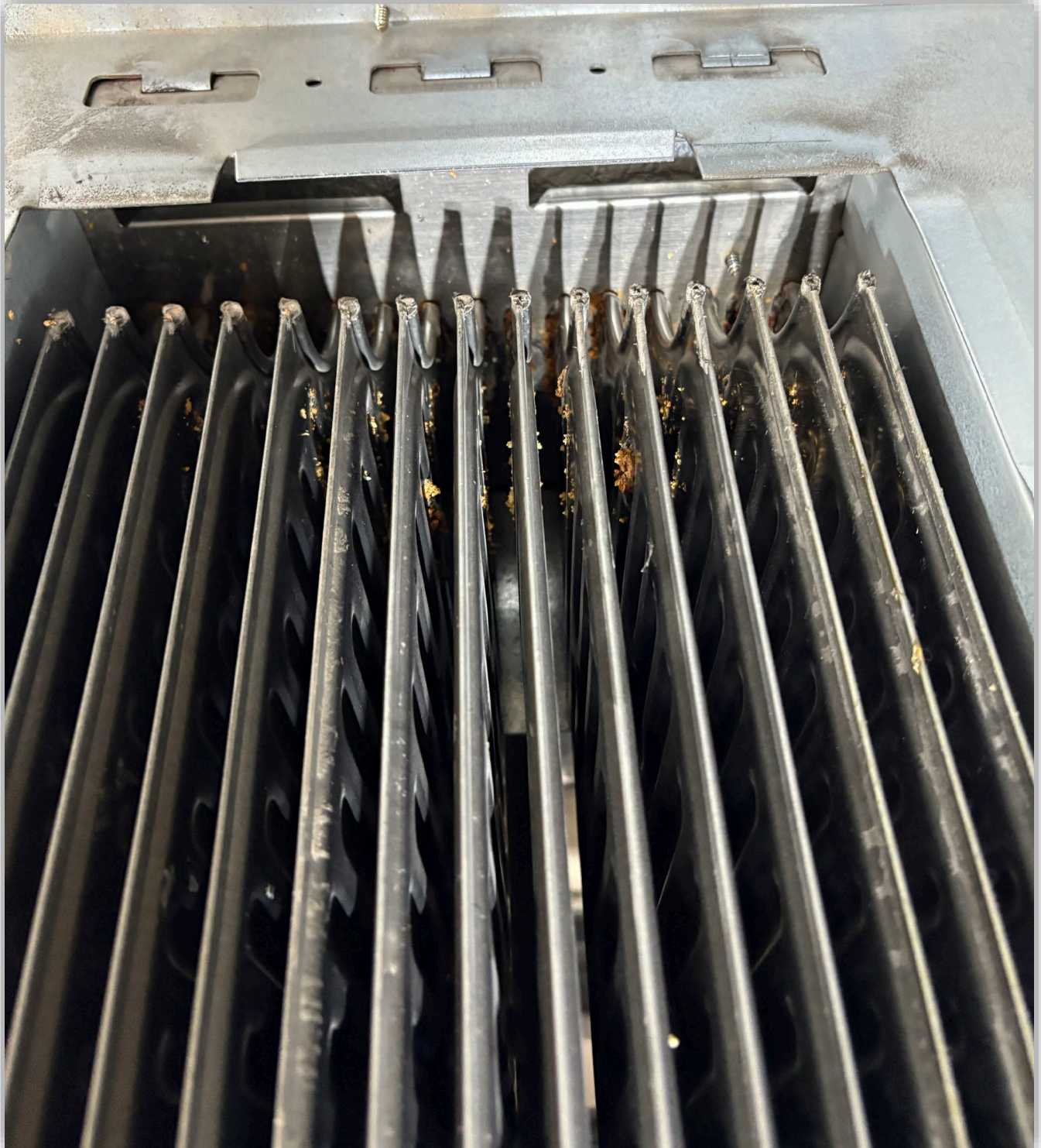
Image 2 – Secondary heat exchanger tubes with exterior corrosion.
