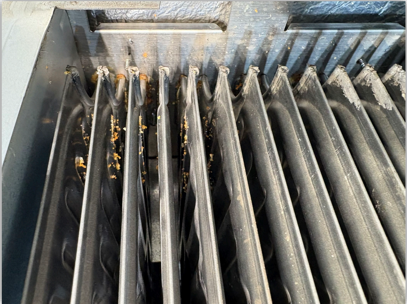
Image 3 – Secondary heat exchanger tubes with exterior corrosion.
