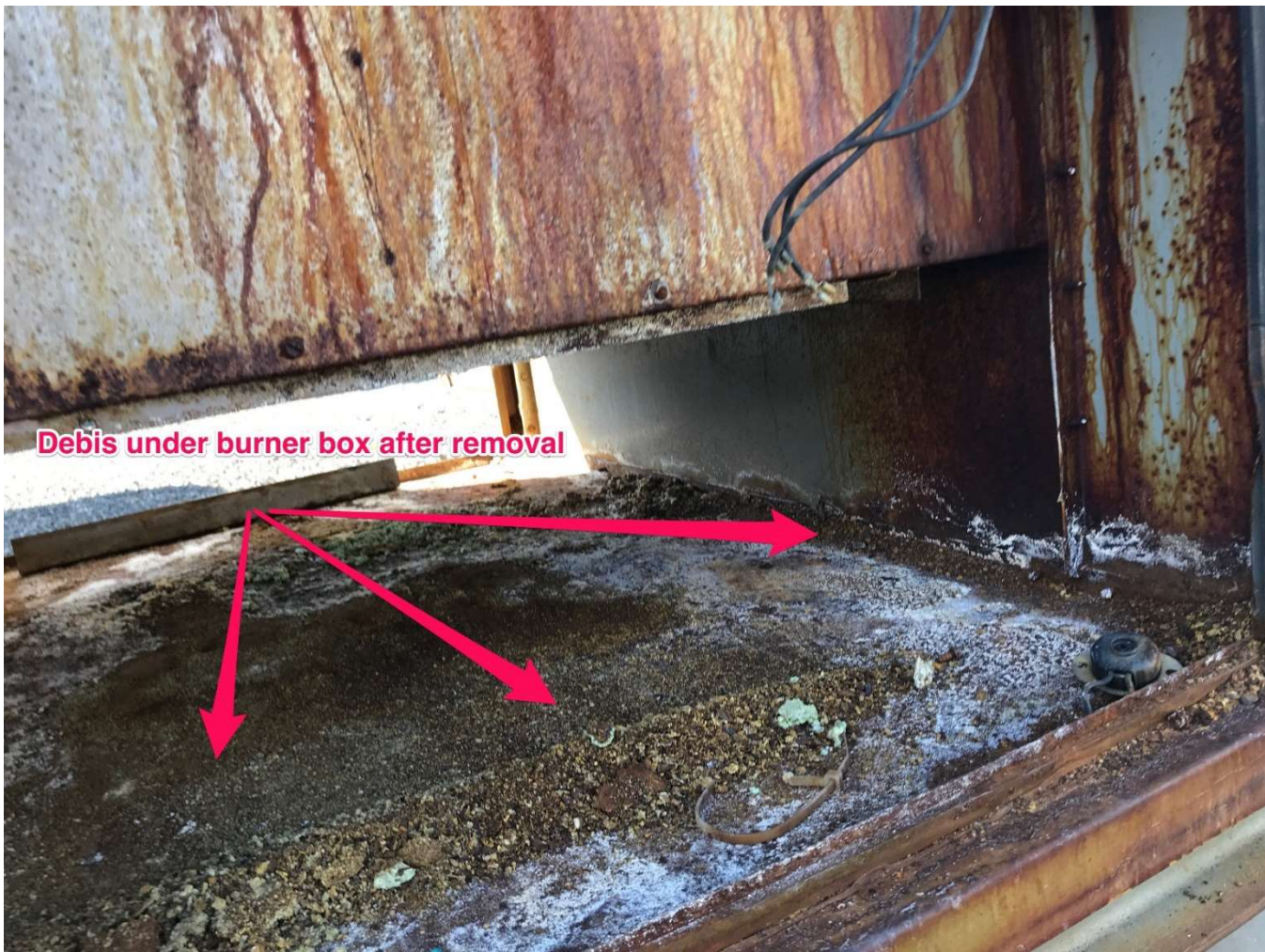
Image #4 Location of burner box after removal from appliance
