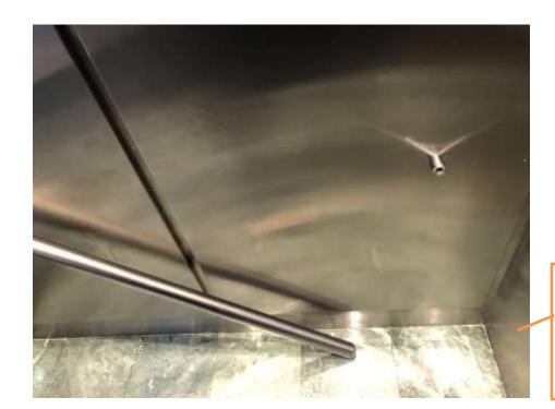
Railing on the floor of the elevator after it was dislodged from the wall
