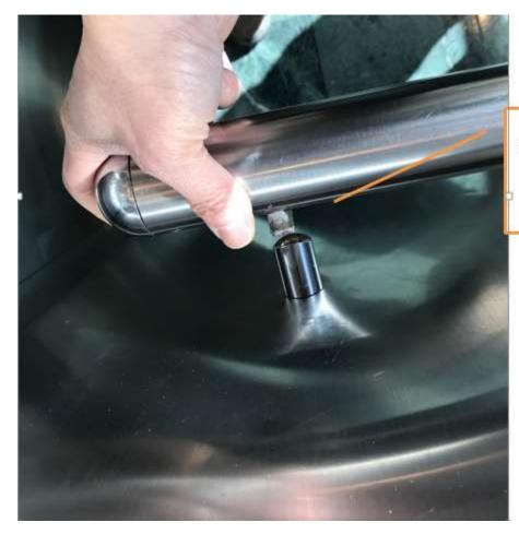
Hand Rail mount and where the railing is fastened with screw
