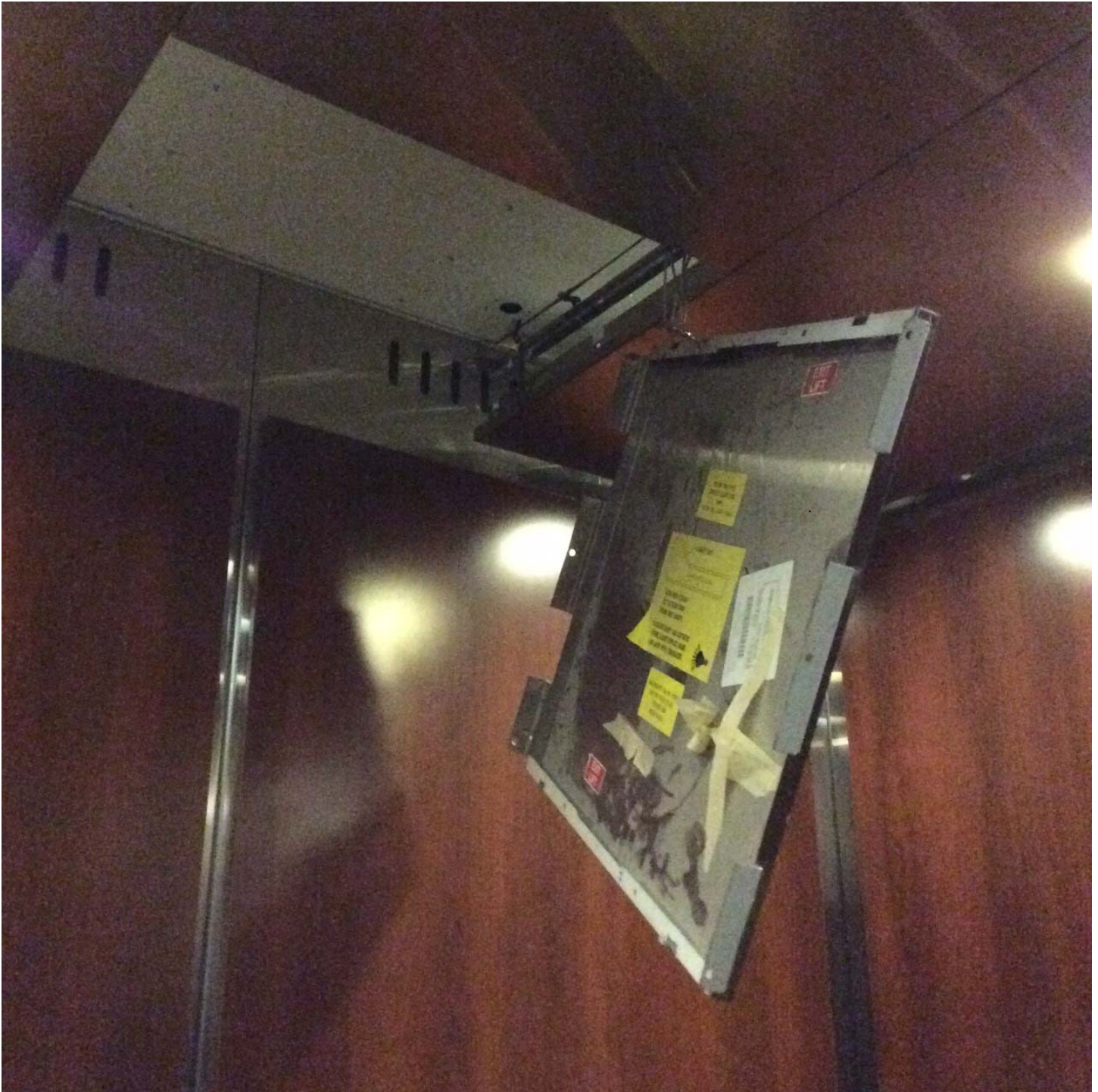
Photo 2. Elevator escape hatch panel securely fastened to elevator cab. Approximately 72 inches from cab floor to lowest edge of escape hatch panel. Photo taken after hatch re-installed.
