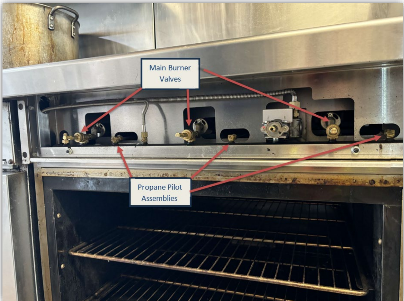
Image 3 – Oven burner valves and pilot assemblies.
