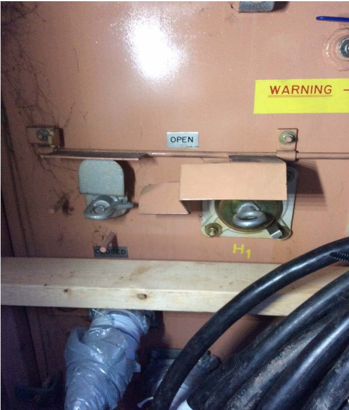
Close up of the High Voltage H1 connection to the draw out bay-o-net fuse.
