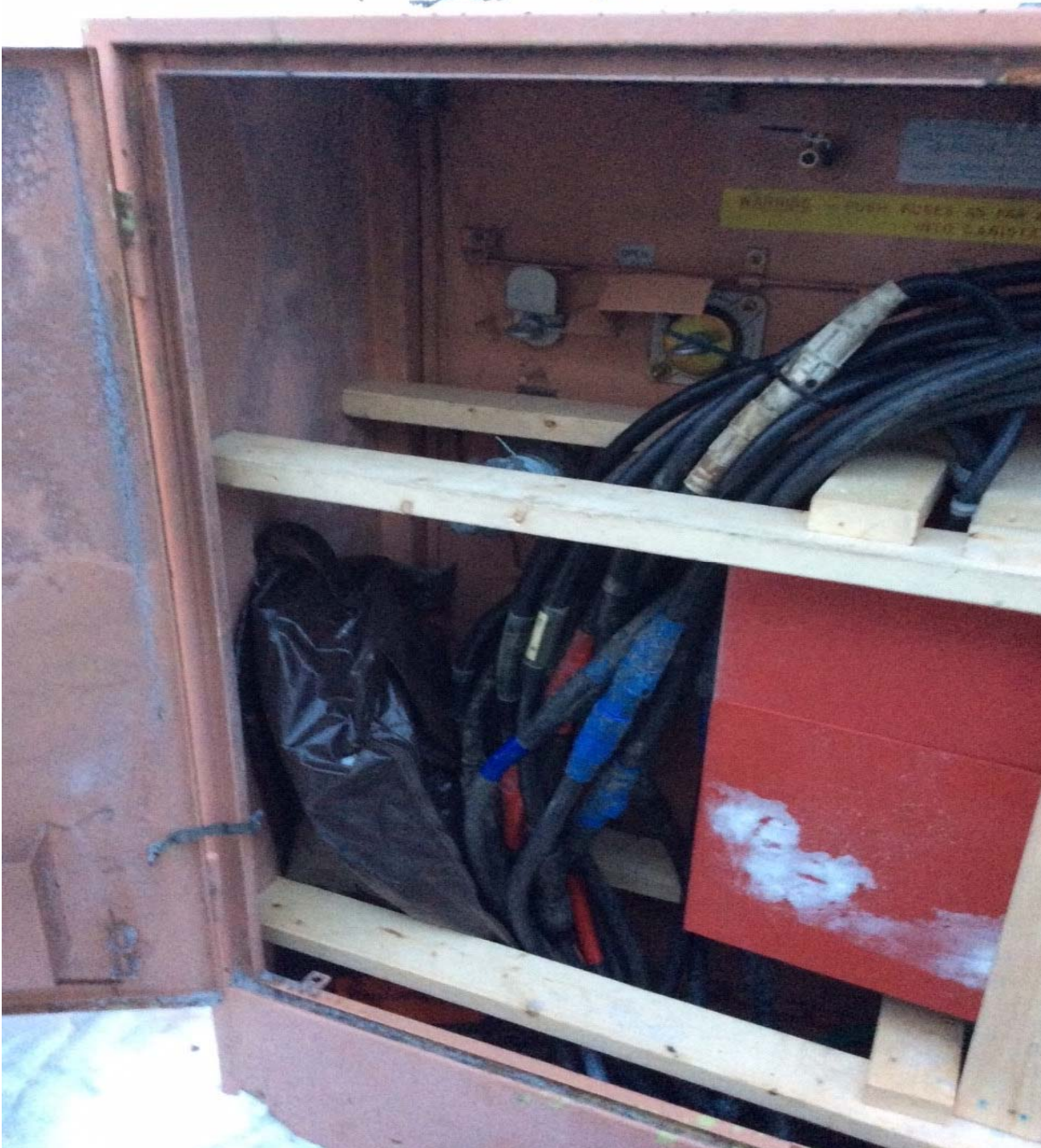
Transformer Compartment, High Voltage connections removed and Low Voltage Connection isolated for temporary Generator connection.
