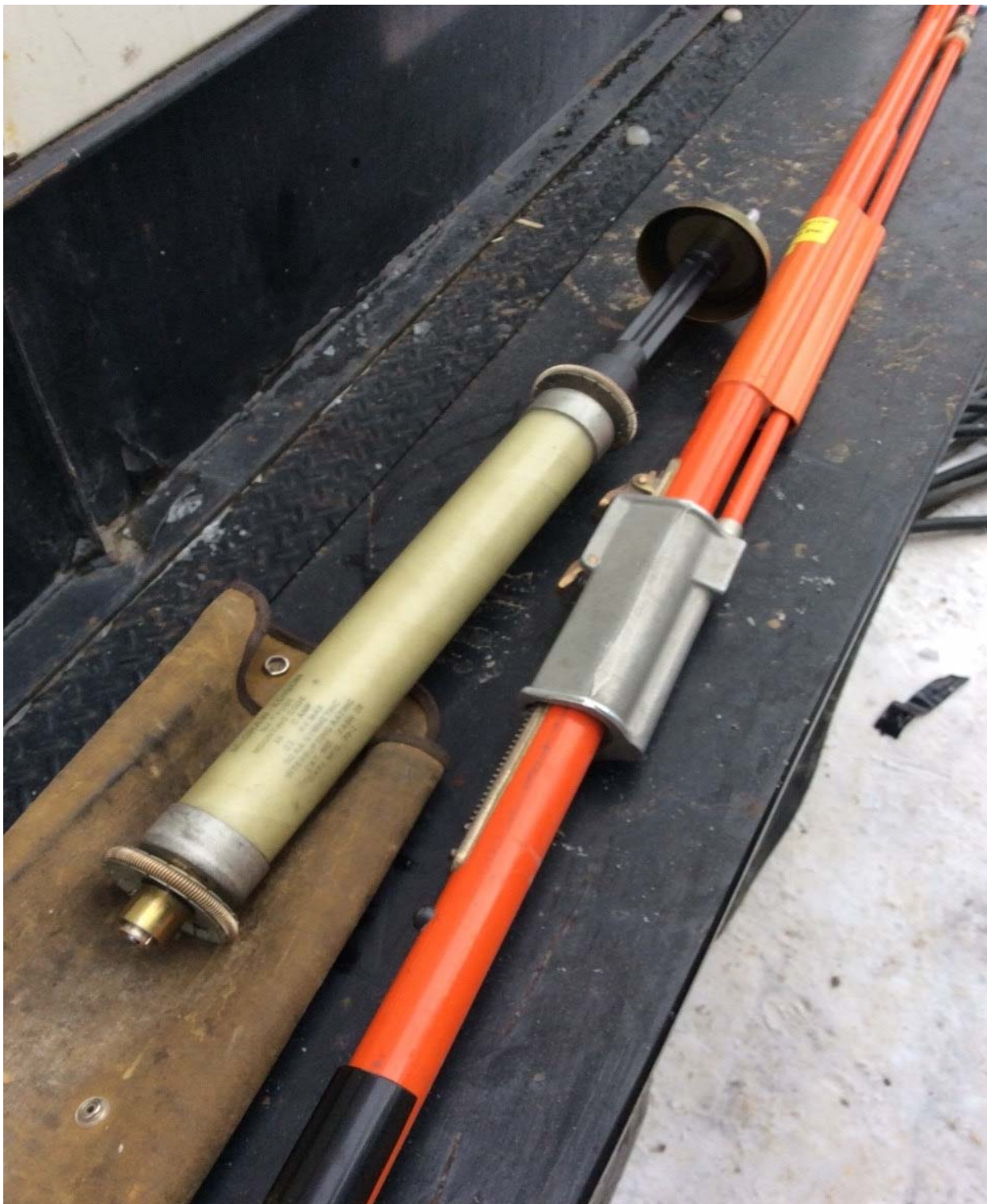
View of Bay-O-Net fuse pulled out of the H1 connection point.
