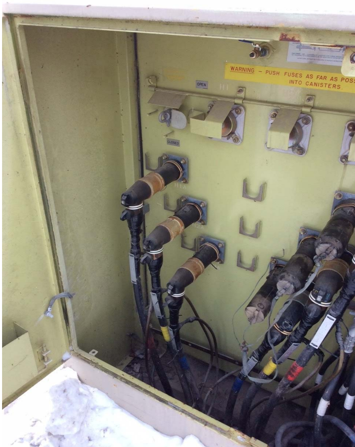
High Voltage connection parked in approved location at the 500KVA Transformer upstream from the blown 500KVA Transformer.
