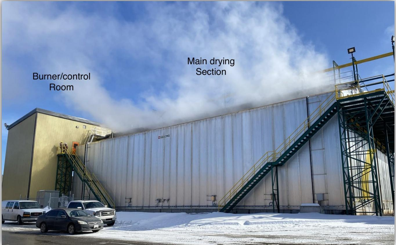
Image 1 – Industrial lumber kiln and attached control building.
