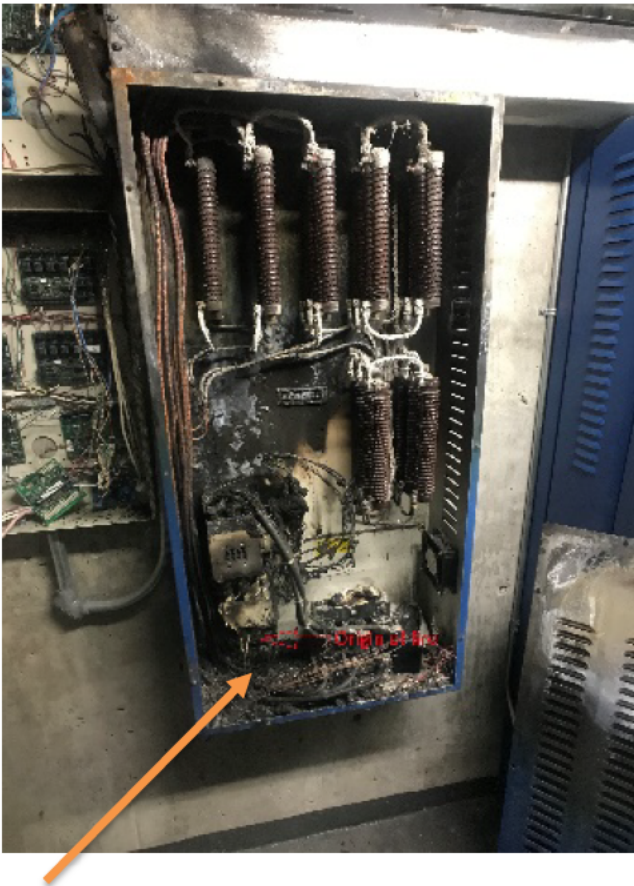
Photo 2 - Origin of the fire just below the motor contactor
