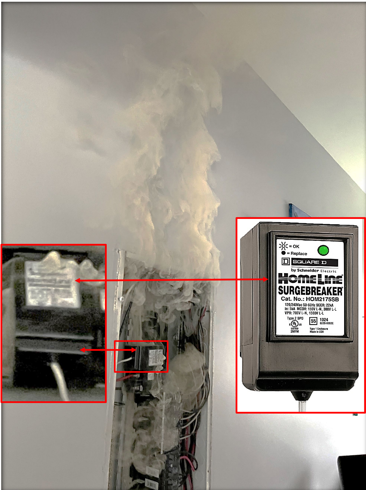
Image 1 – Main panel board with smoke billowing out, SPD, and example SPD on right.
