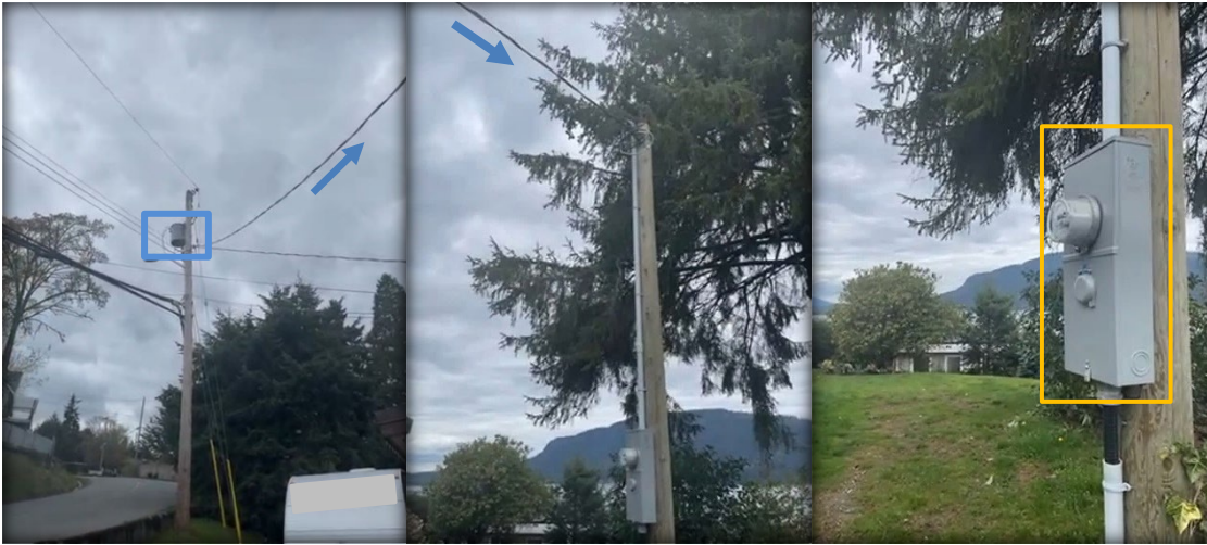
Image 3a,b,c – Supply transformer (blue rectangle), overhead supply line (blue arrows), and combination meter base with circuit breaker (orange rectangle).
