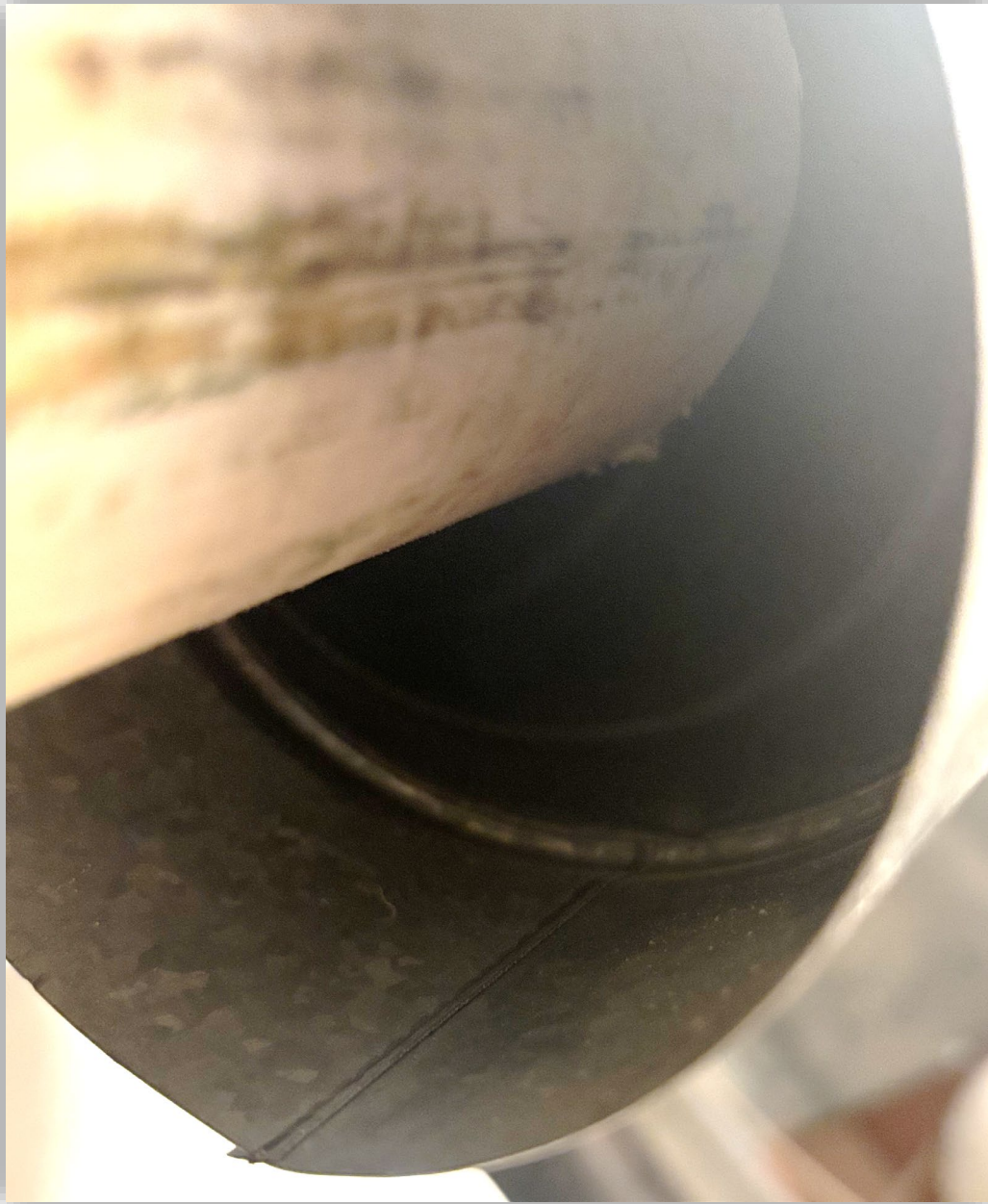
Image 2 - The end of the 2" plastic pipe is visible inside the 4" metal vent. There is no adapter made for this installation, and the installer did not attempt to seal the gap between the two venting systems. This allowed carbon monoxide from the water heater to spill into the residence instead of being directed to the outside.
