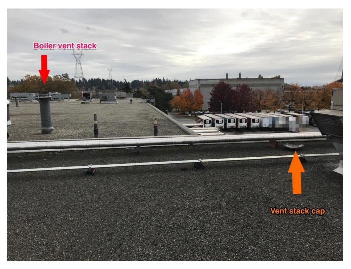
Image 6 - Location of vent cap after it was blown off the boiler vent stack by the explosion
