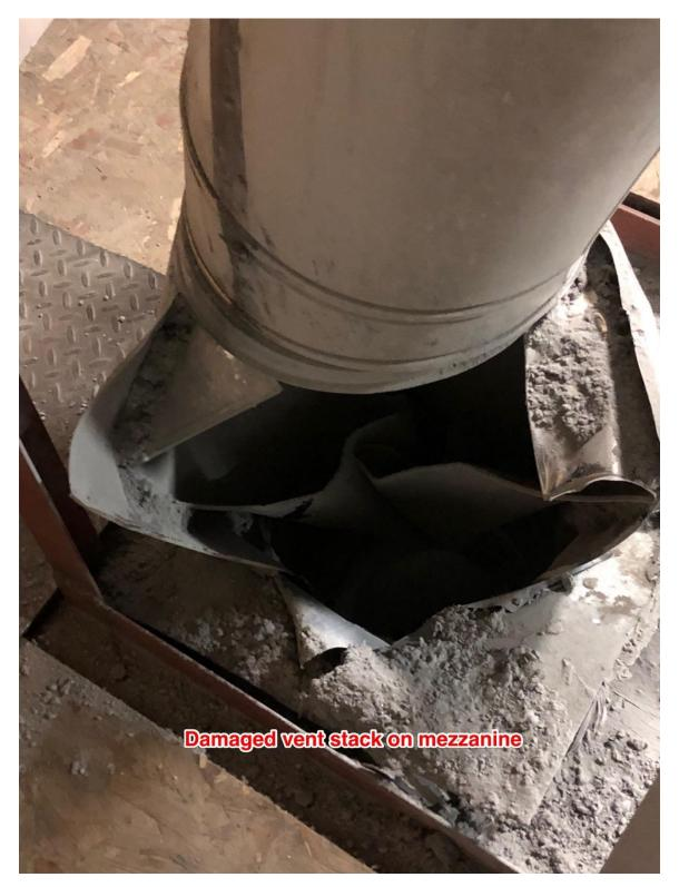
Image 5 - Boiler vent stack at mezzanine above boiler room
