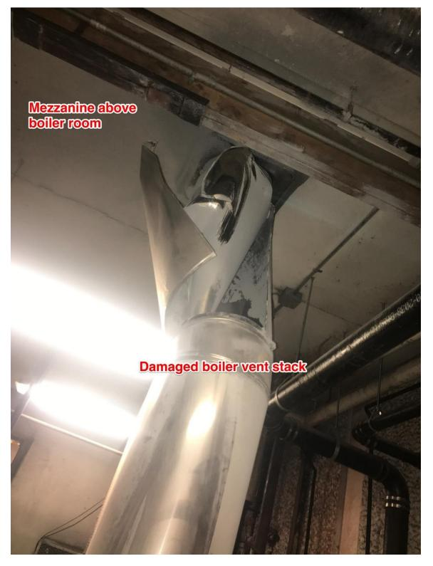
Image 4 - Boiler vent stack above boiler
