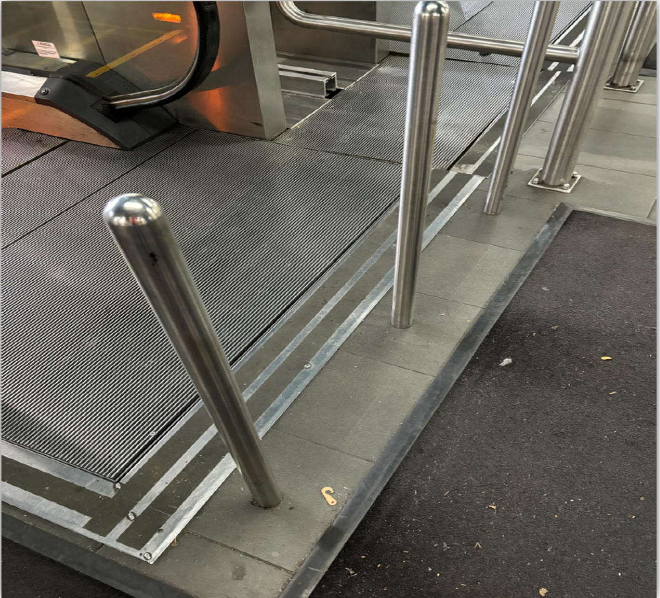
Image 1 – Bollards to prevent carts on escalator.
