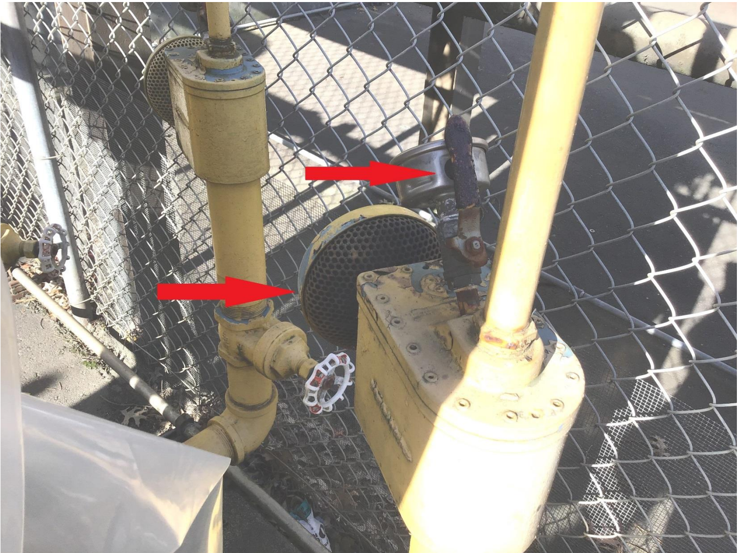
Figure 3. Close-up of leaking mixer, again note the burned handle and blackened receiver screen.
