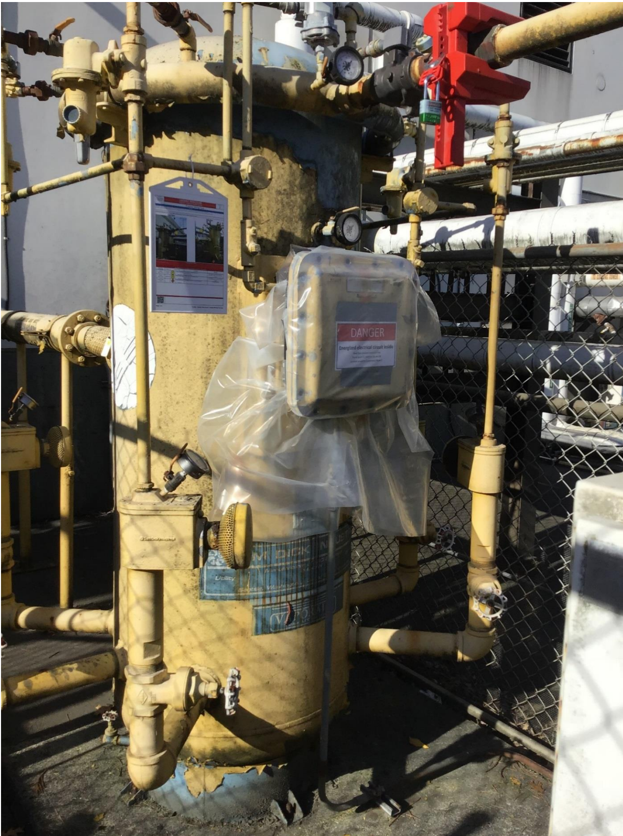
Figure 1. Propane air mixer on day of investigation.
