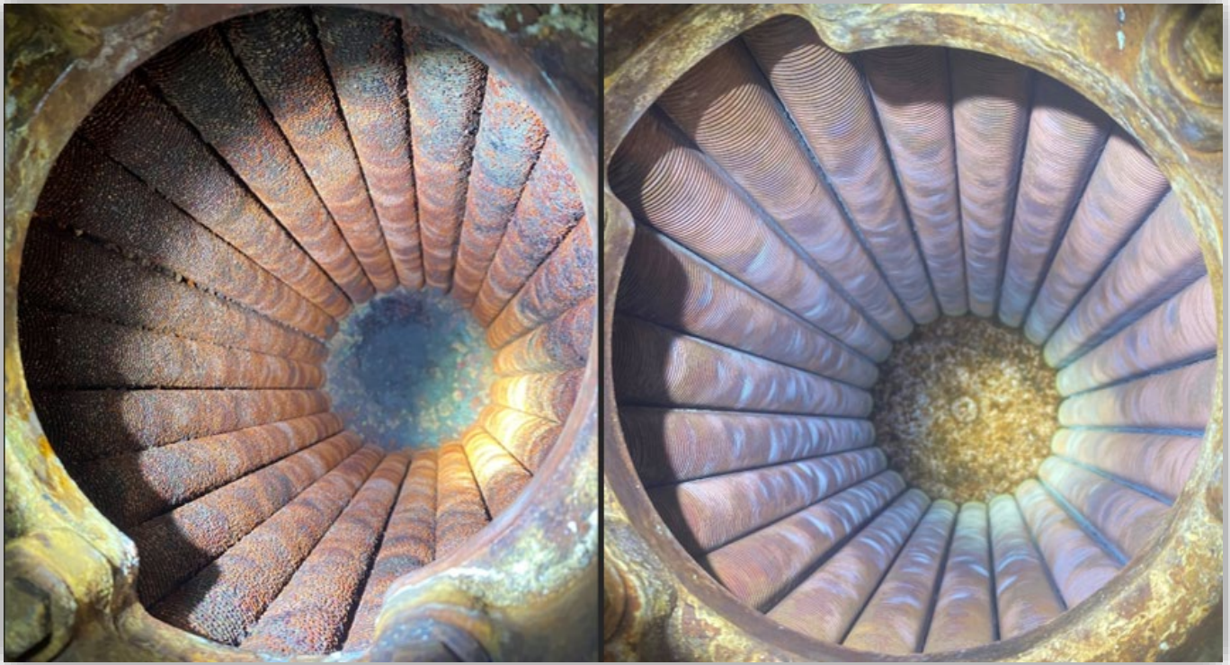
Image 5 – Comparison of the dirty and plugged heat exchanger of Boiler #1 (Left) to relatively clean heat exchanger of Boiler #2 (Right).
