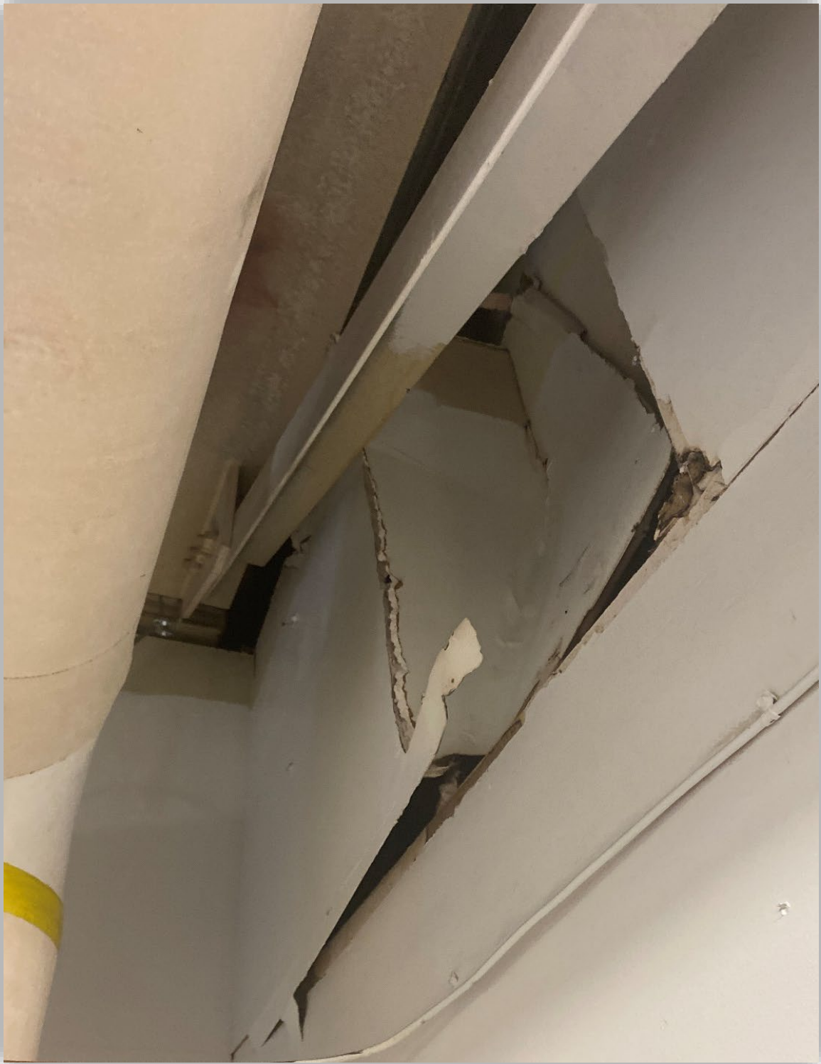
Image 3 – Damaged drywall at ceiling of mechanical room.
