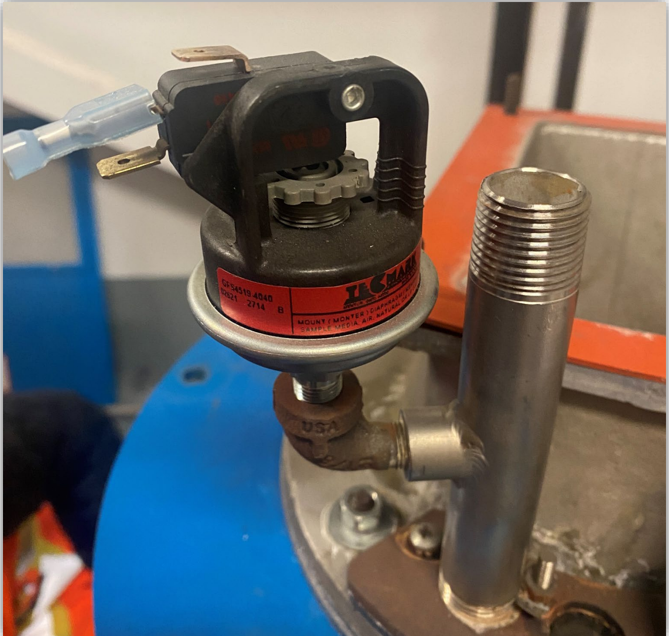
Image 8 – High exhaust backpressure switch installed on boiler with a black iron street elbow. (Image taken during disassembly with other components and wiring removed).
