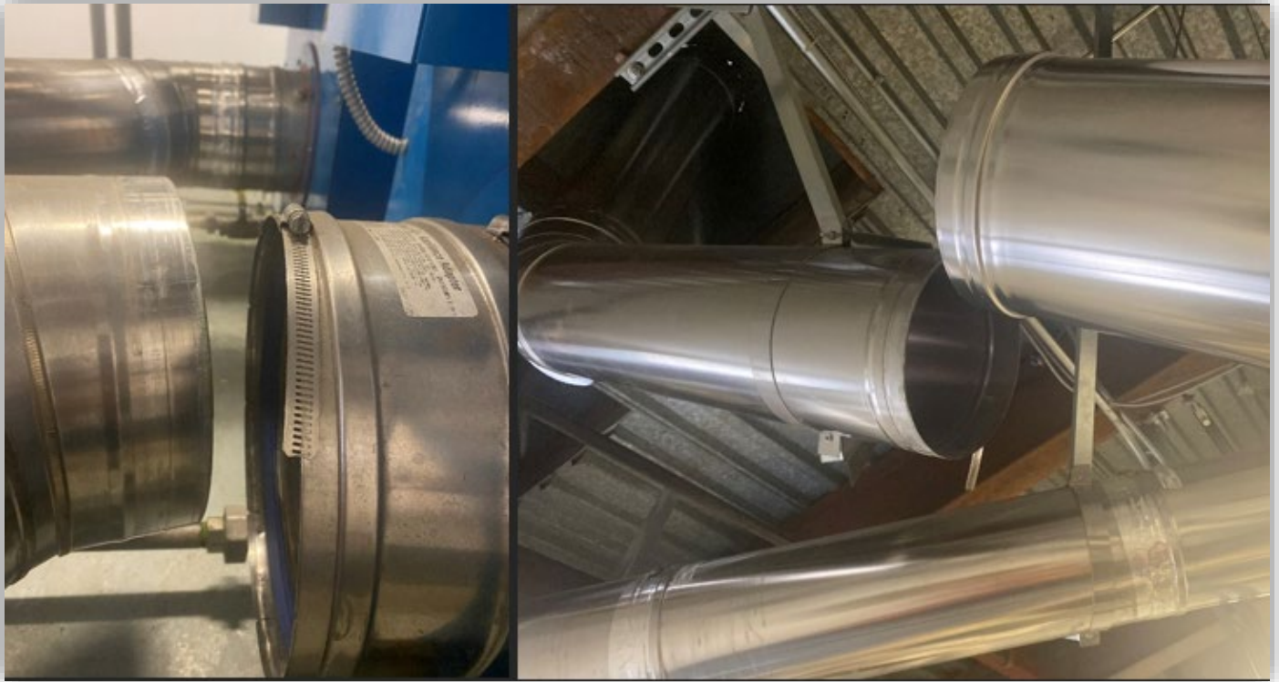
Image 4 – Dislodged venting components from Boiler #1 after explosion.
