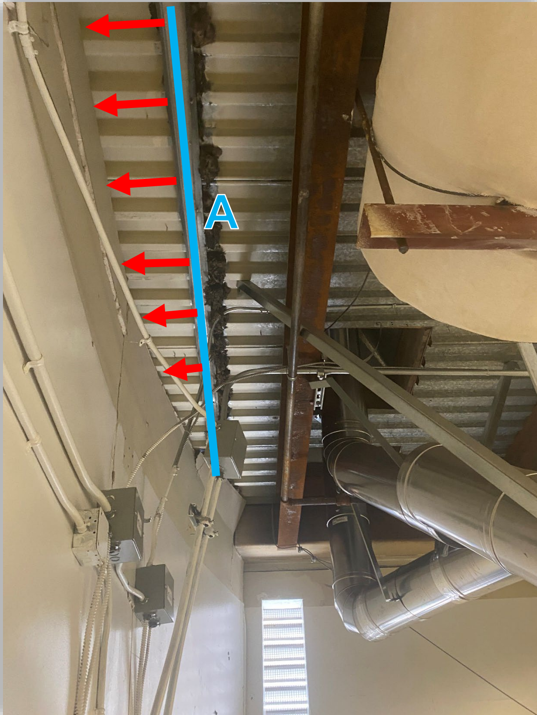
Image 2 – Damaged wall of mechanical room. [A] line indicated original location of the wall and the arrows show the amount the wall was pushed in by the explosion.
