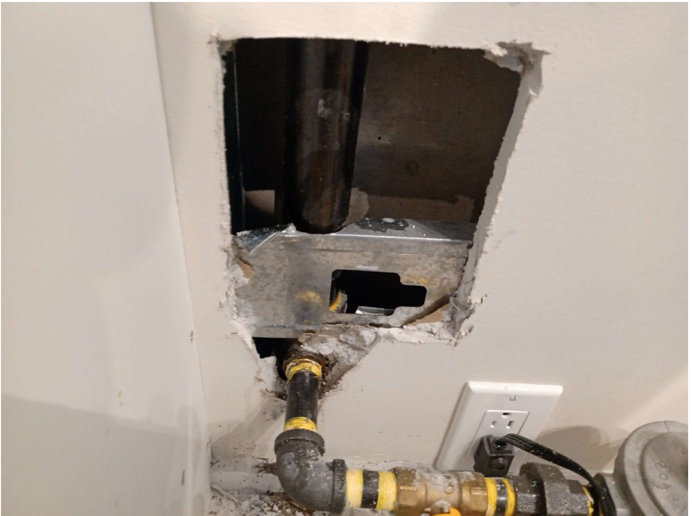
Figure 3 - Gas pipe in the wall
