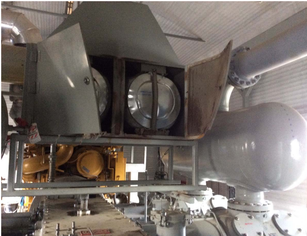
K-440 Compressor intake – may have contributed to ignition of vapour cloud - notice damaged doors
