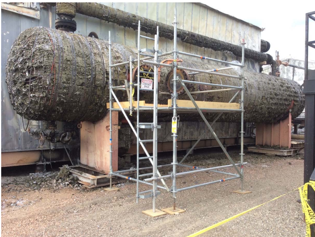
V-665 Low Temperature Separator – exterior fire damaged.
