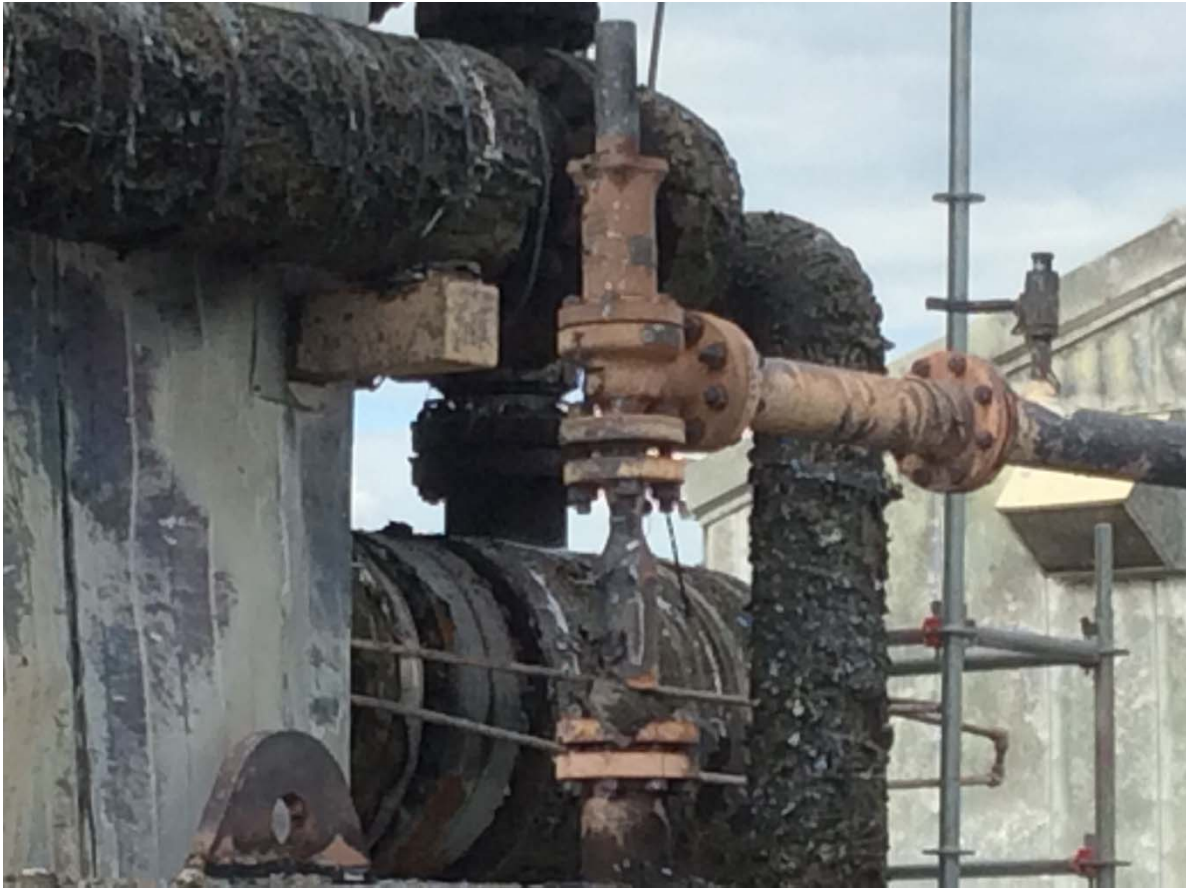
V-665 Low Temperature Separator – Safety Relief Valve
