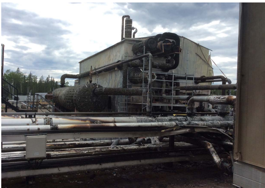
V-665 (horizontal Low pressure separator on left) - Z-650 Refrigeration Building (on right)
