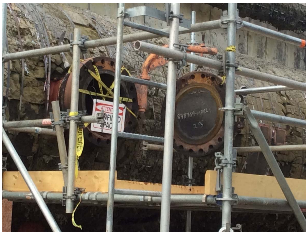
V-665 Low Temperature Separator – Inspection Nozzle in opened during investigation by Owner
