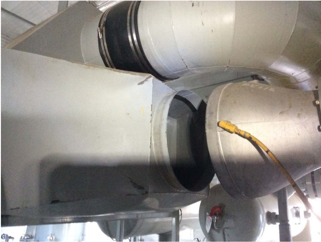
K-440 Compressor damage on rear side of air intake assembly
