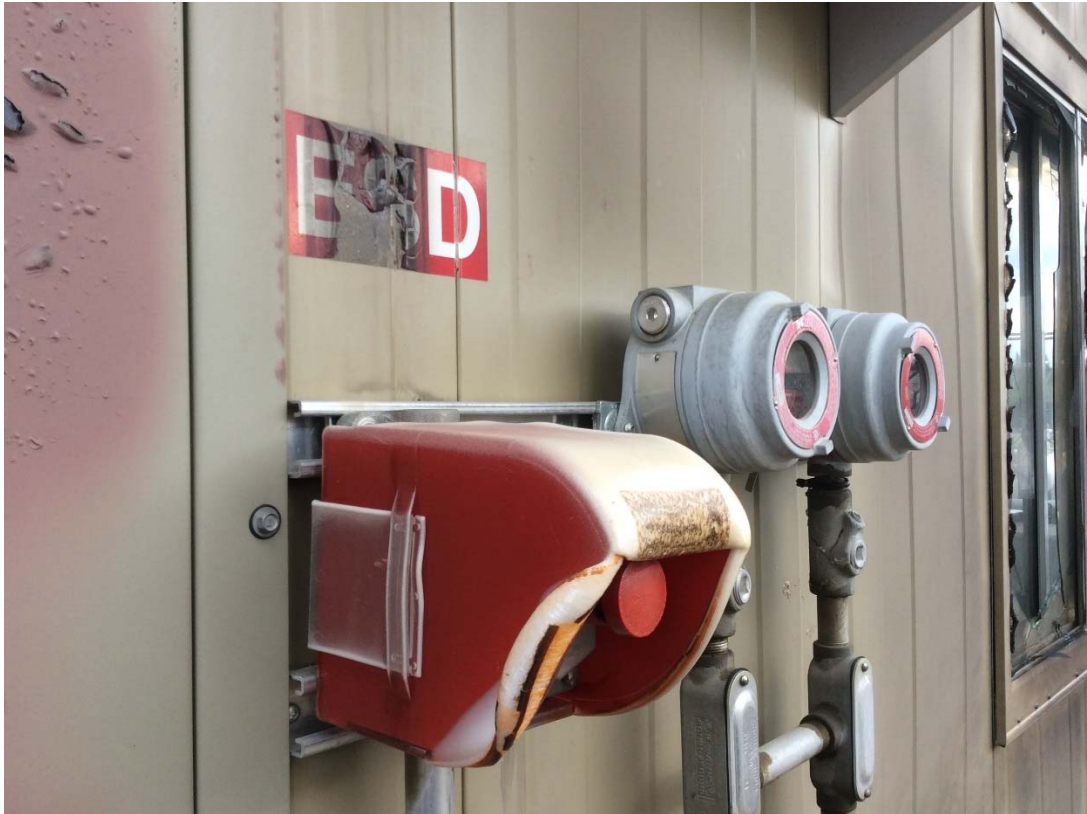
K-440 Compressor building melted ESD button
