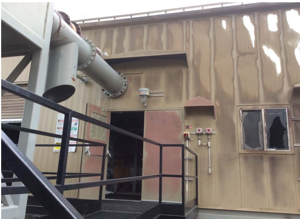
K-440 Compressor building melted paint, windows and exterior steel wall
