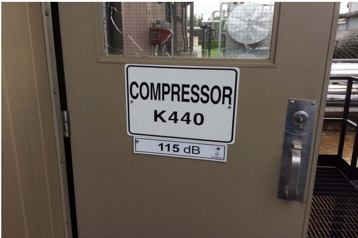
K-440 Compressor doorway – Note broken safety glass
