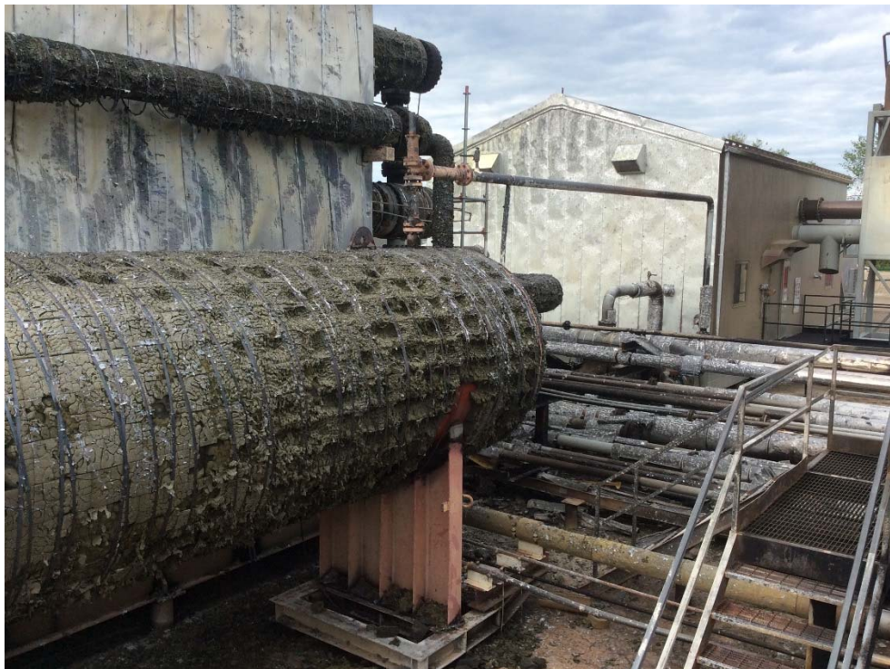
V-665 Low Temperature Separator – Safety Relief Valve on right end at 12 o'clock position
