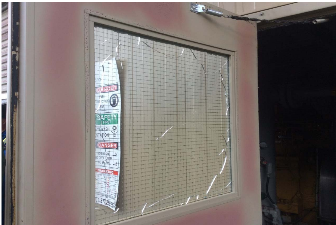
K-440 building door- note heat pattern around broken window
