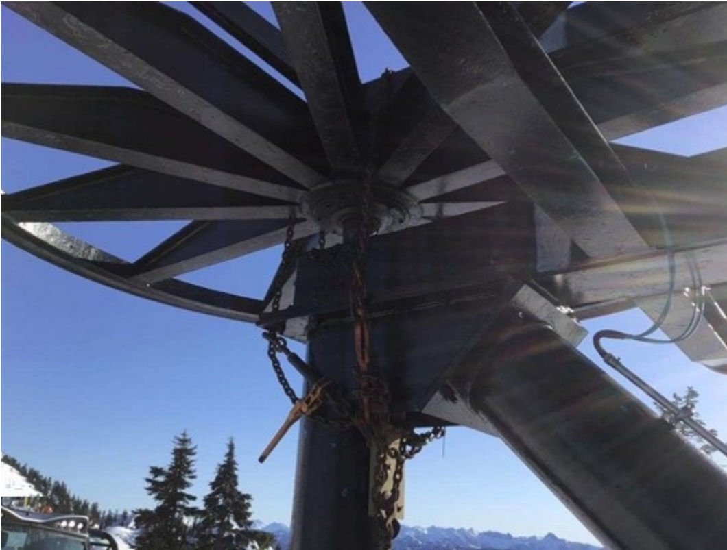
Photo 5, Bull wheel (chains and load binders installed to prevent further lifting of the bull wheel assembly).
