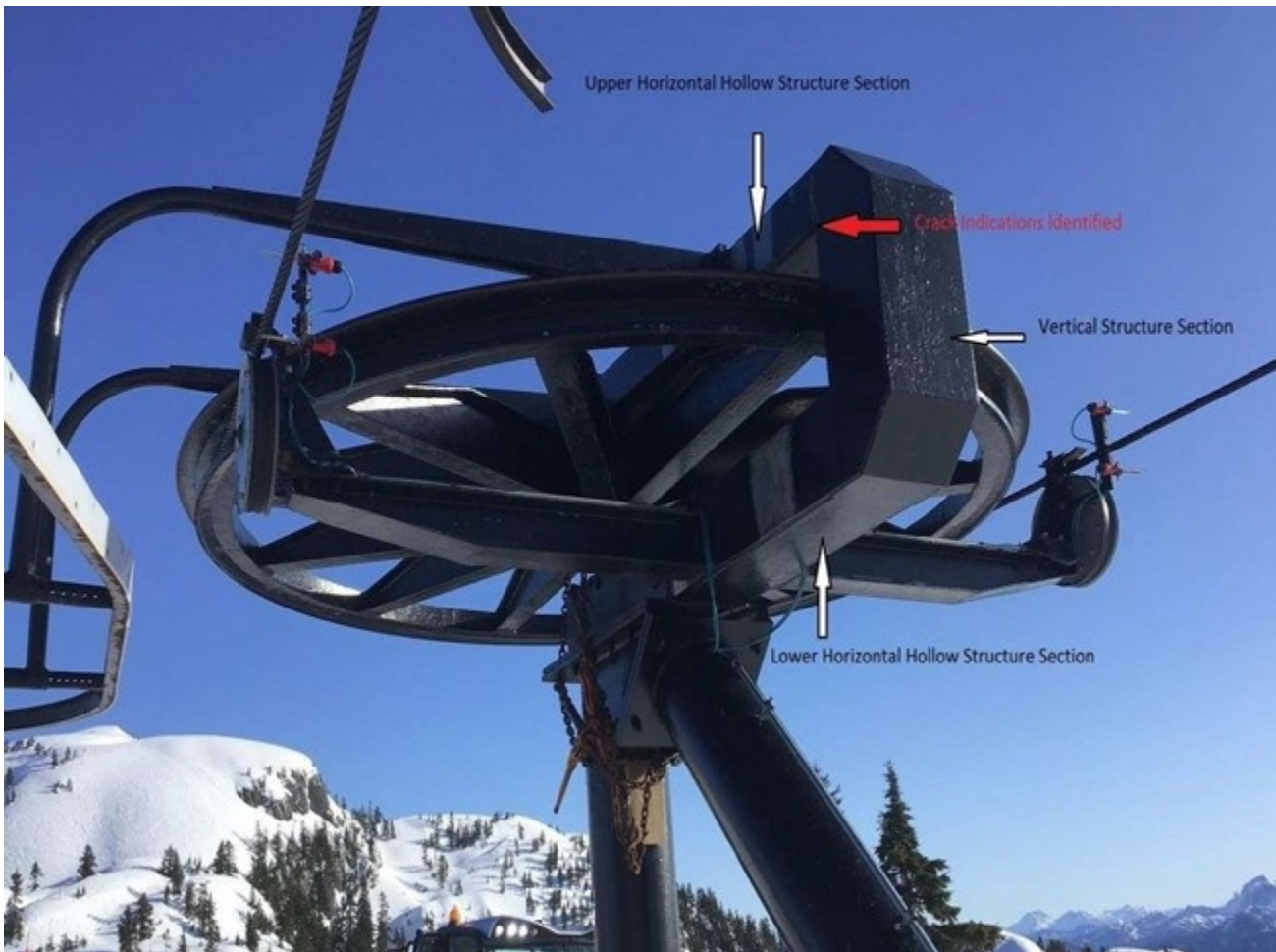
Photo 2, Bull Wheel F Frame Labeled, Guide Sheaves Shown in Photo
