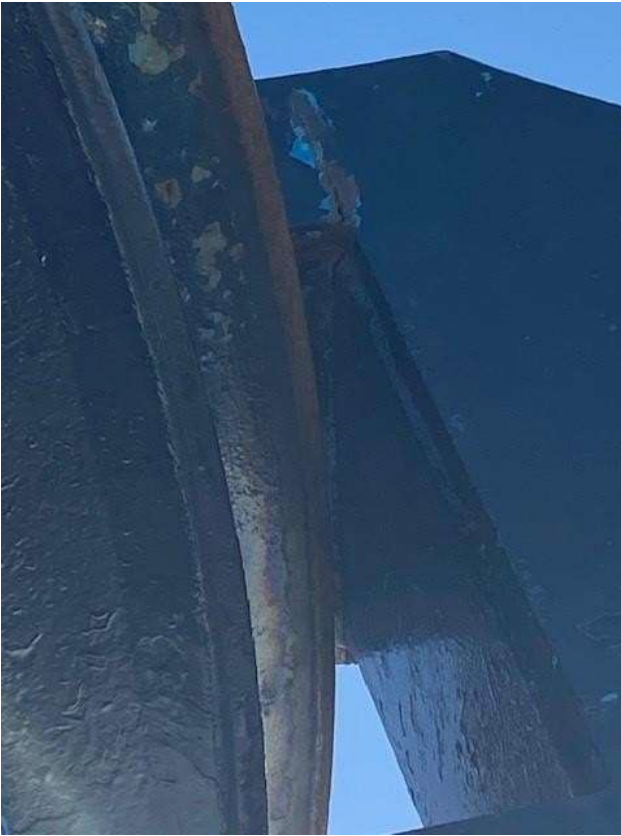
Photo 3, Crack Indication in F Frame. See Photo 2.
