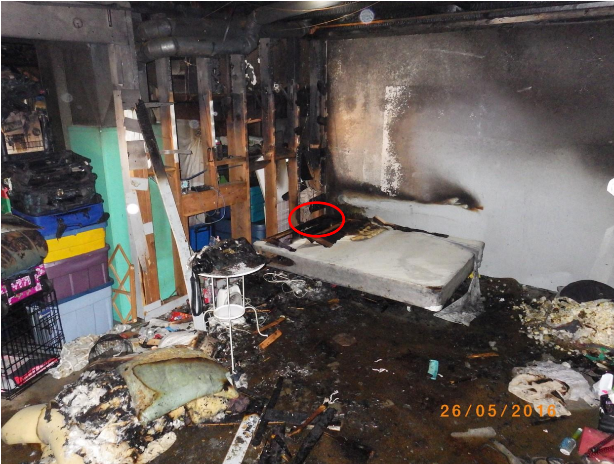
Figure 2 – Basement bedroom and area of origin determined by fire department investigators (red outline). Box spring only - the mattress was removed by fire fighters at the time of the fire.
