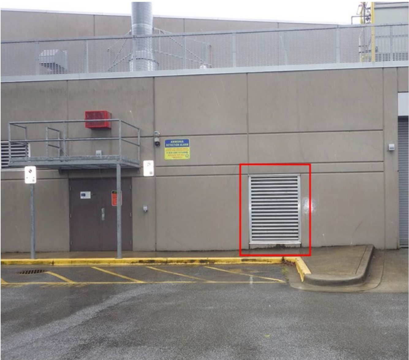
Image 8 - Red box showing air intake to this machinery room which ammonia entered during the release.
