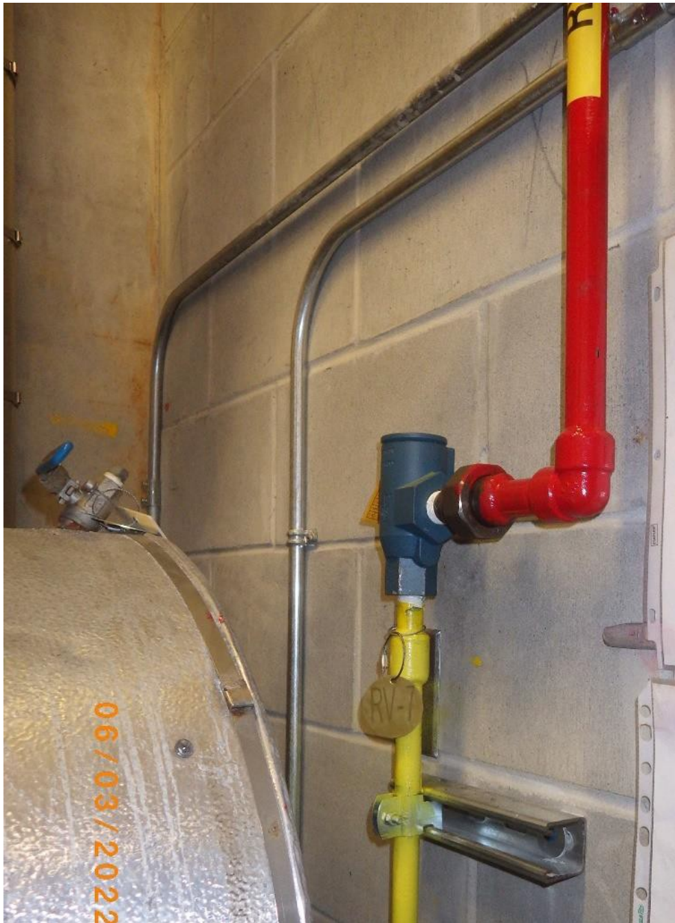
Image 6 - Oil pot and the attached safety valve, the one that opened discharging liquid ammonia to the outside vent stack.
