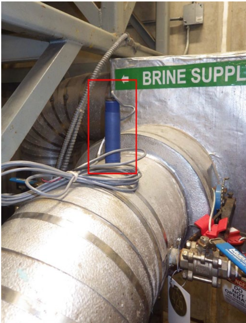
Image 4 – Red box showing newly installed pH sensor in the brine discharge piping.
