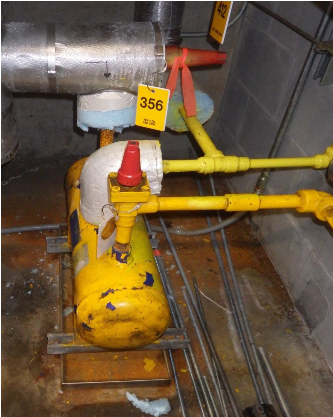
Image 5 - Oil pot located on the machinery room floor beside the chiller.
