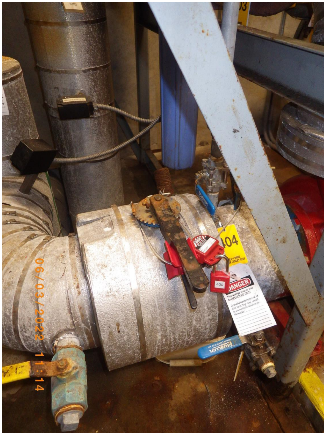
Image 3 - Brine pump suction valve with scissor clip and lock, (Closed position) as found after incident.
