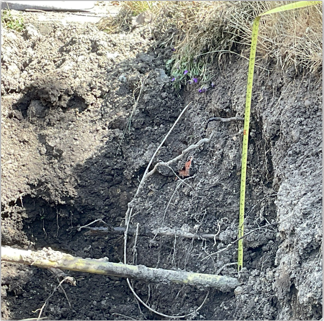
Image 3 - Gas line to surface to depth (22 inches) measured at location post gas line strike.
