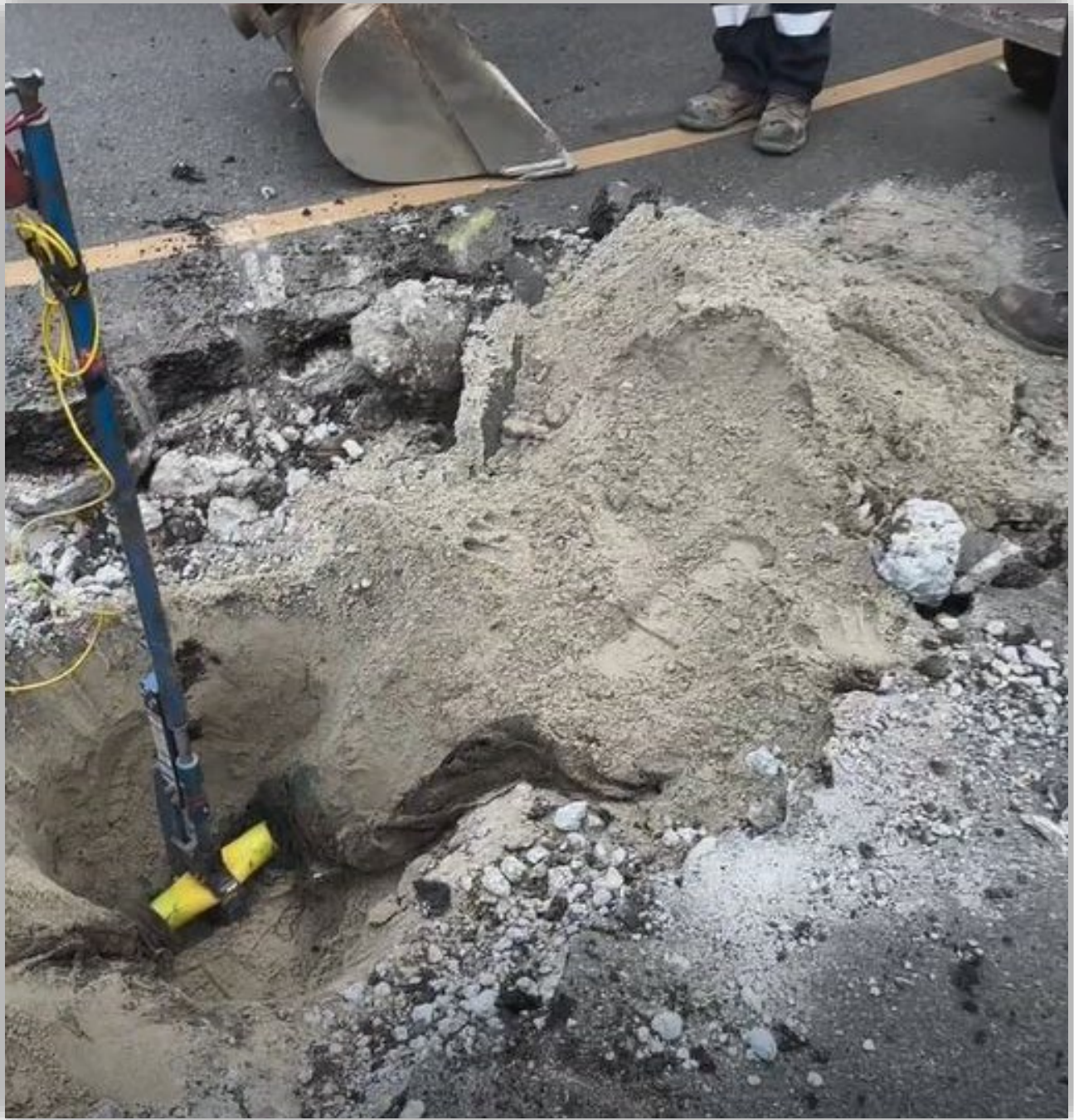
Image 4 - Post incident gas line clamped off at street by Fortis.
