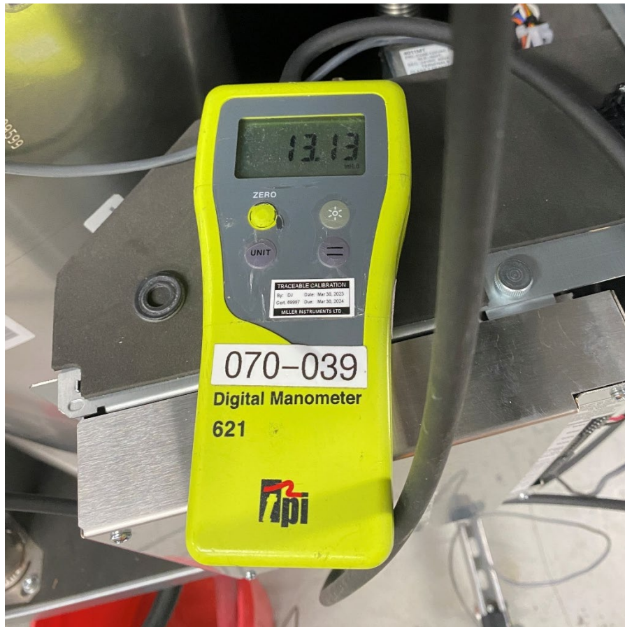
Image 3 – Inlet gas pressure measurement.
