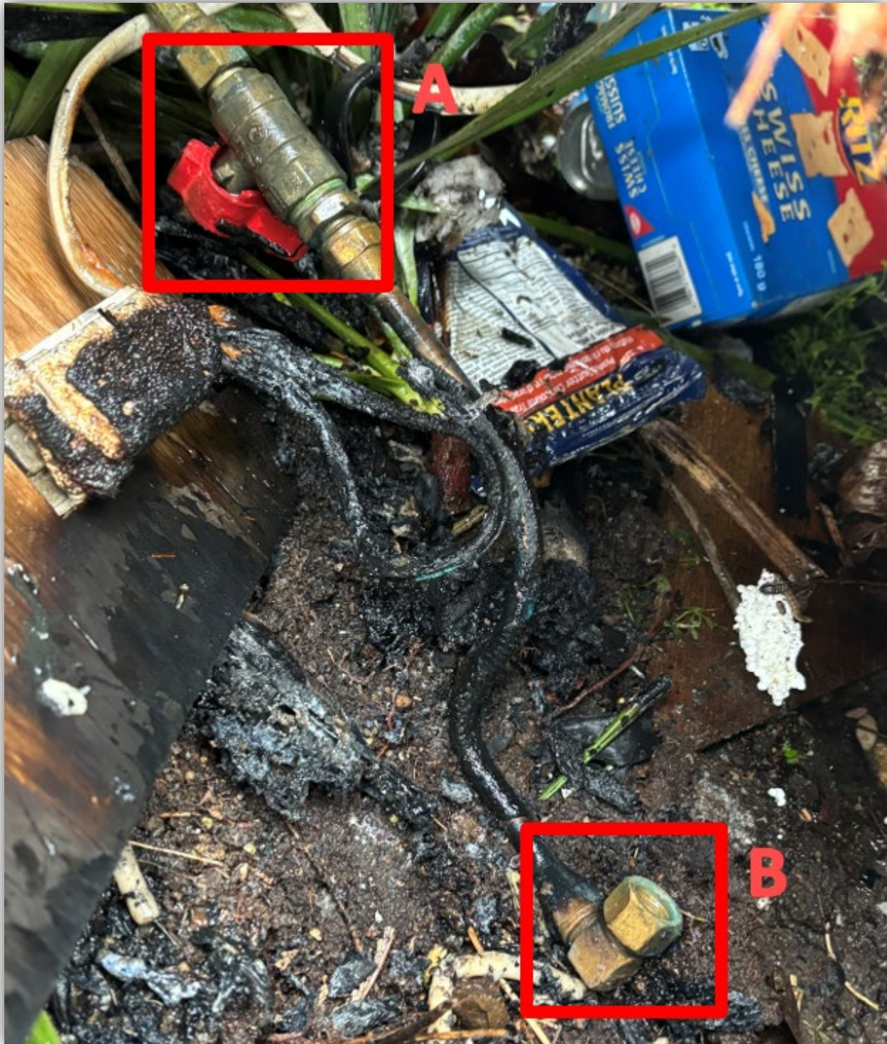
Image 8 – Original fridge gas line with partially open gas valve (A) and unplugged end (B).
