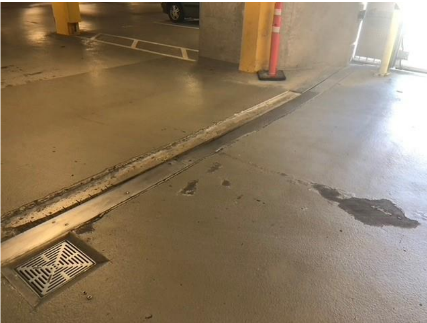
Figure 2 : Rubber expansion joint with steel flanges installed
