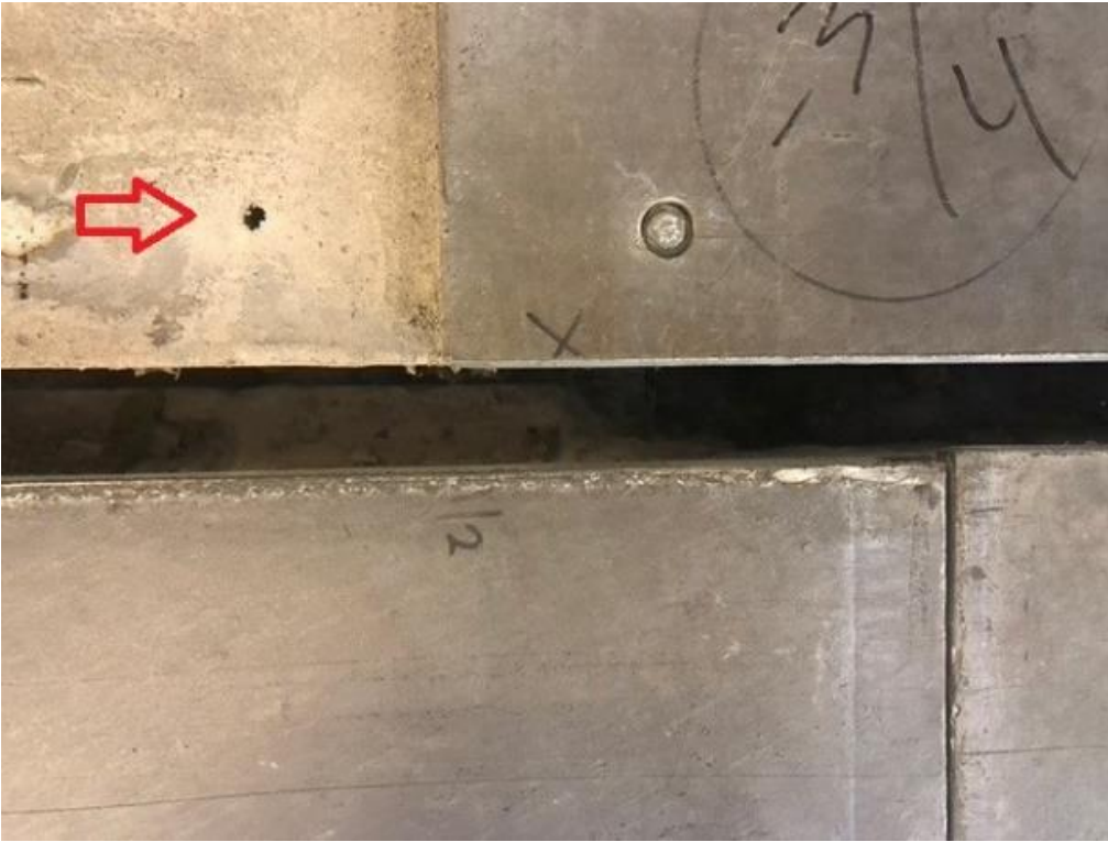
Figure 1 1/4inch hole drilled 6inches deep into the fire pump armoured cable in the concrete slab
