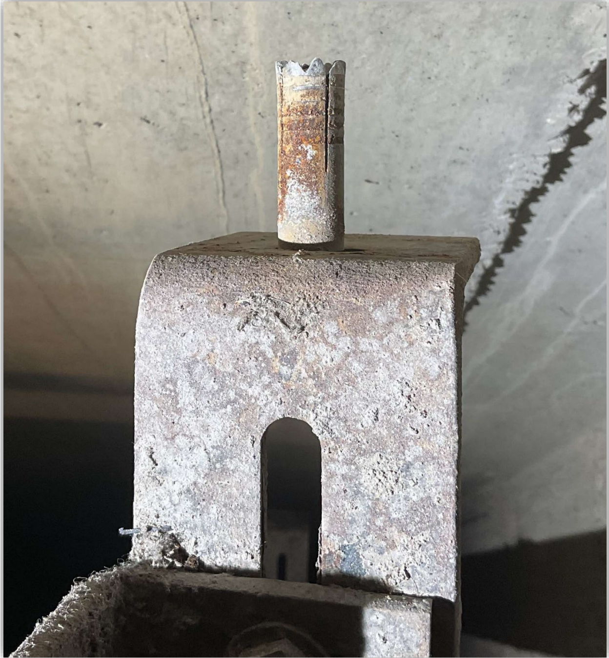
Image 7 – Counterweight guide rail bracket from the 5th floor with concrete anchor insert that had pulled out from the wall.
