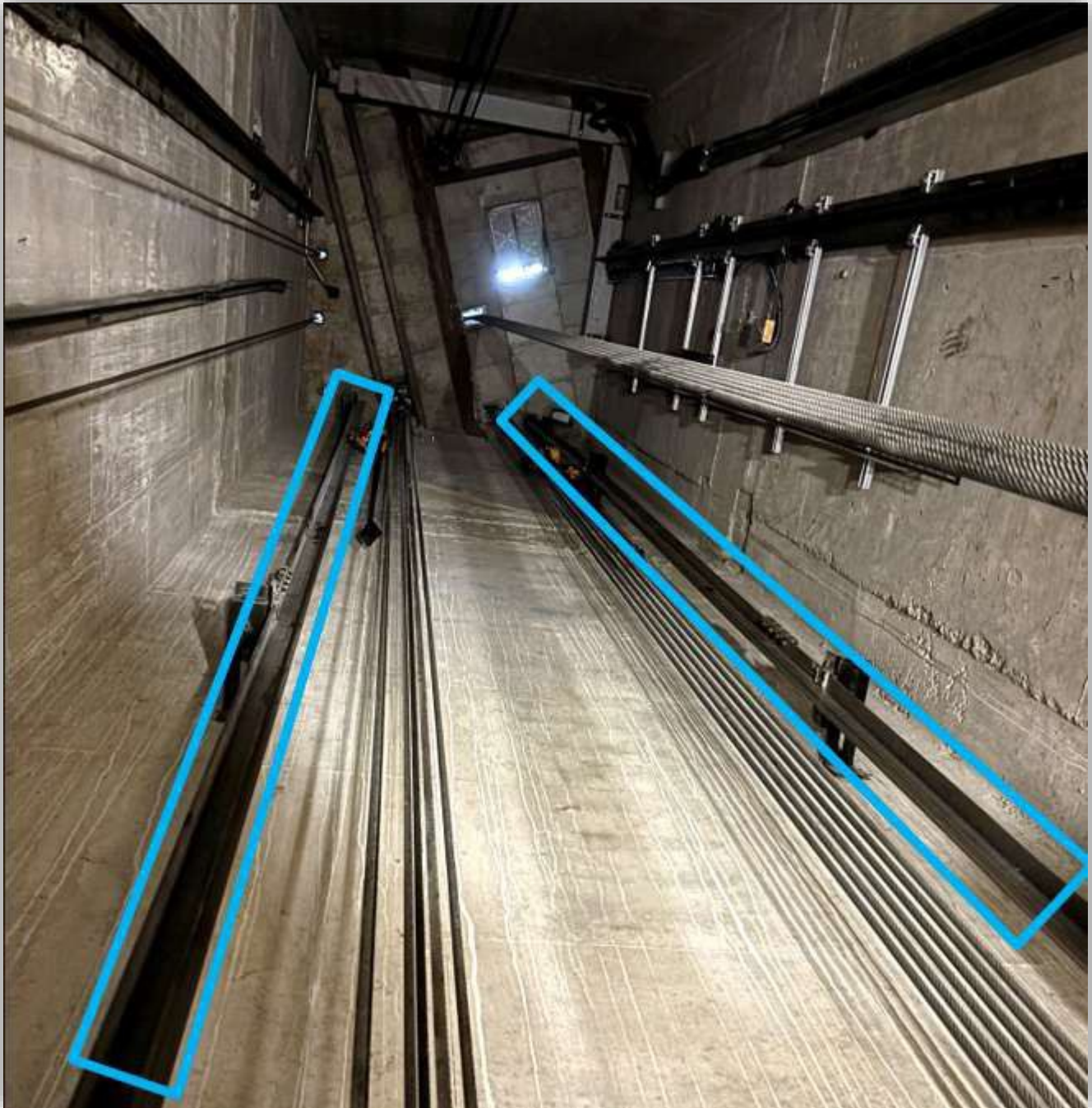
Image 1 – Top of hoistway. [Boxes] The counterweight guide rails.
