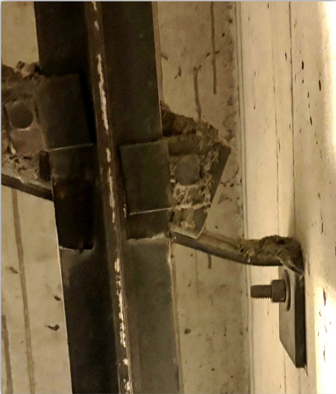
Image 4 – Another counterweight guide rail bracket bent up from contact with the traveling counterweight.
