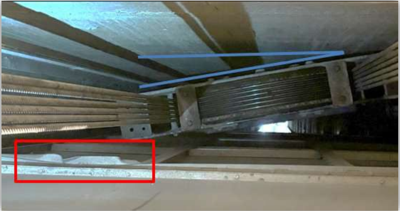
Image 5 – Free hanging elevator counterweight derailed from guide rails showing angle away from wall [lines] and location of damage on elevator car [box].
