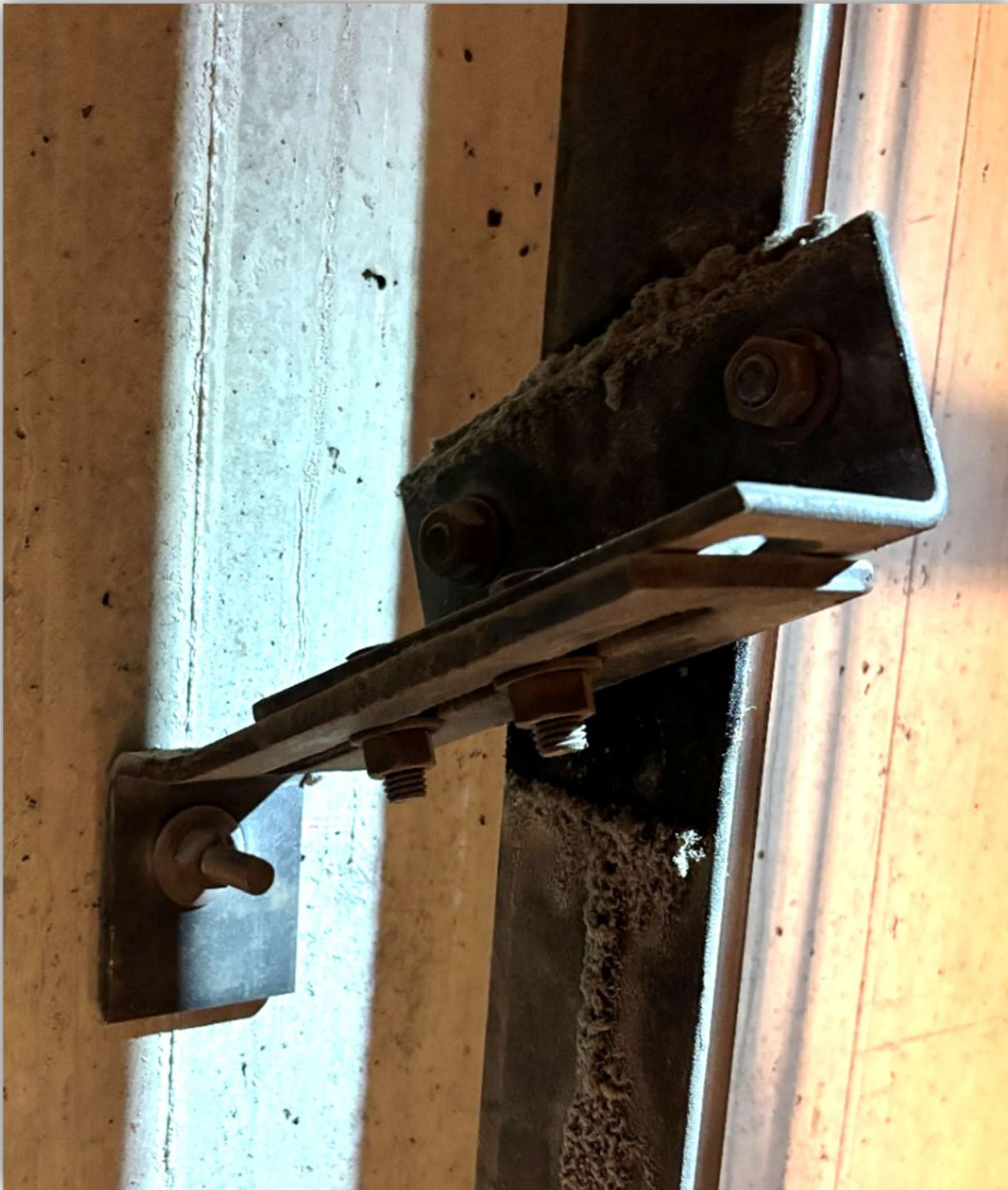
Image 3 - Counterweight guide rail bracket bent up from contact with the traveling counterweight.
