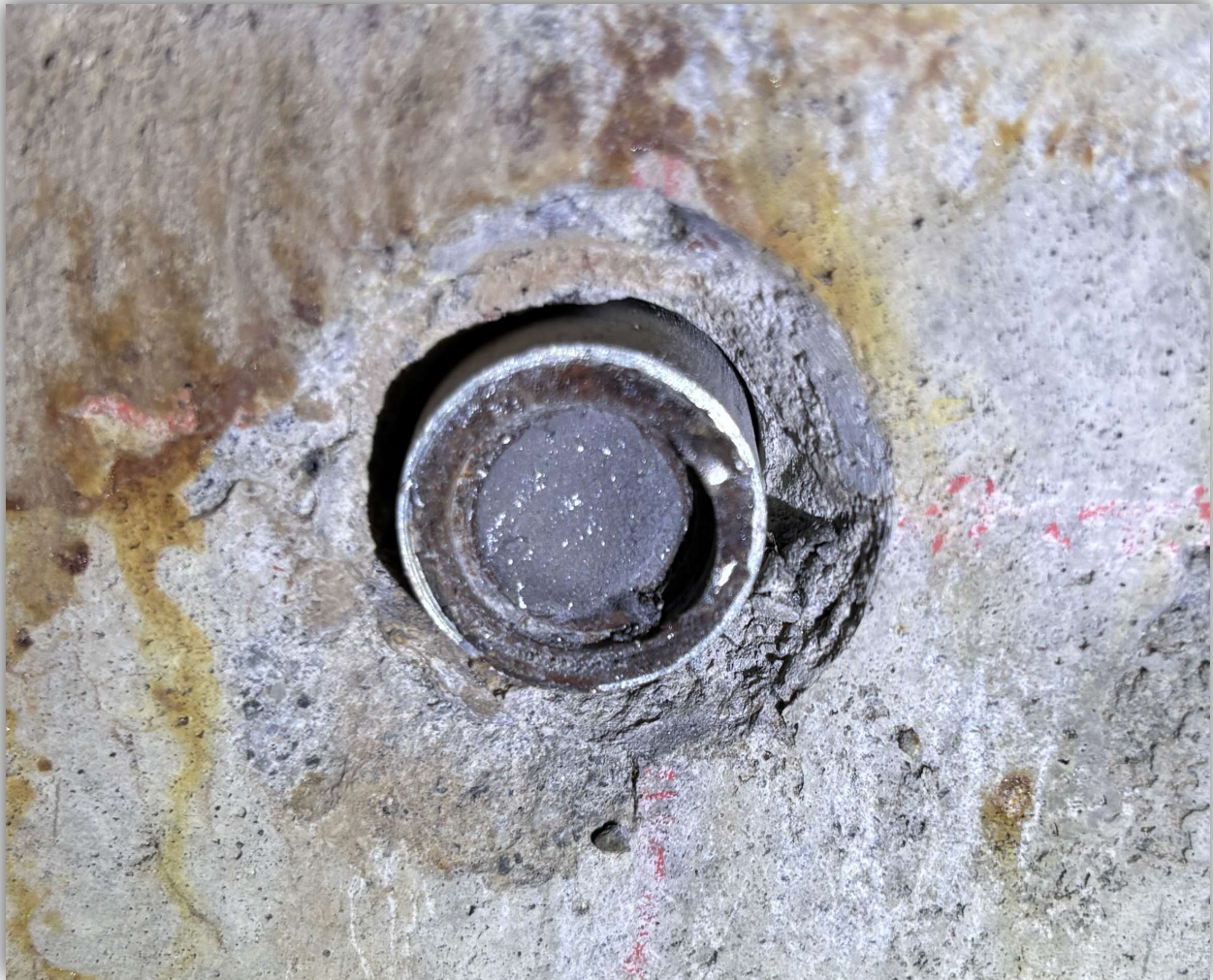
Image 9 – Counterweight guide rail bracket anchor location on the 4th floor with a portion of the broken threaded rod still in the insert.
