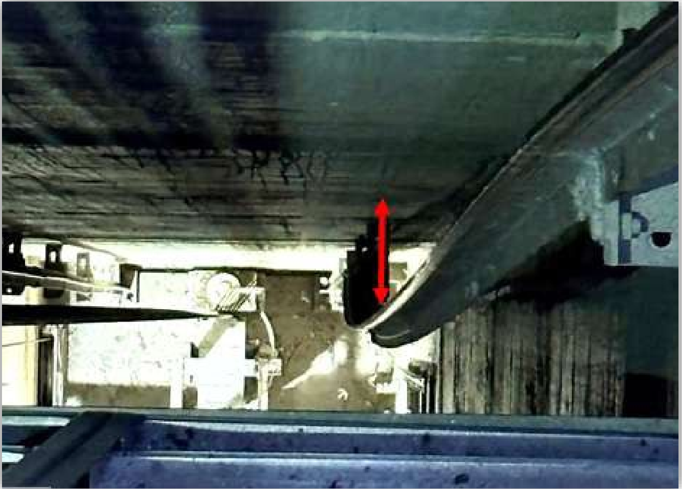
Image 6 - Counterweight guide rail bowed away from the wall.
