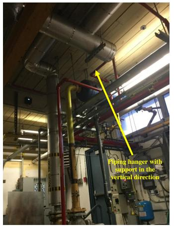
Figure 5: No supports in the horizontal direction on the suction piping above compressor #2.
