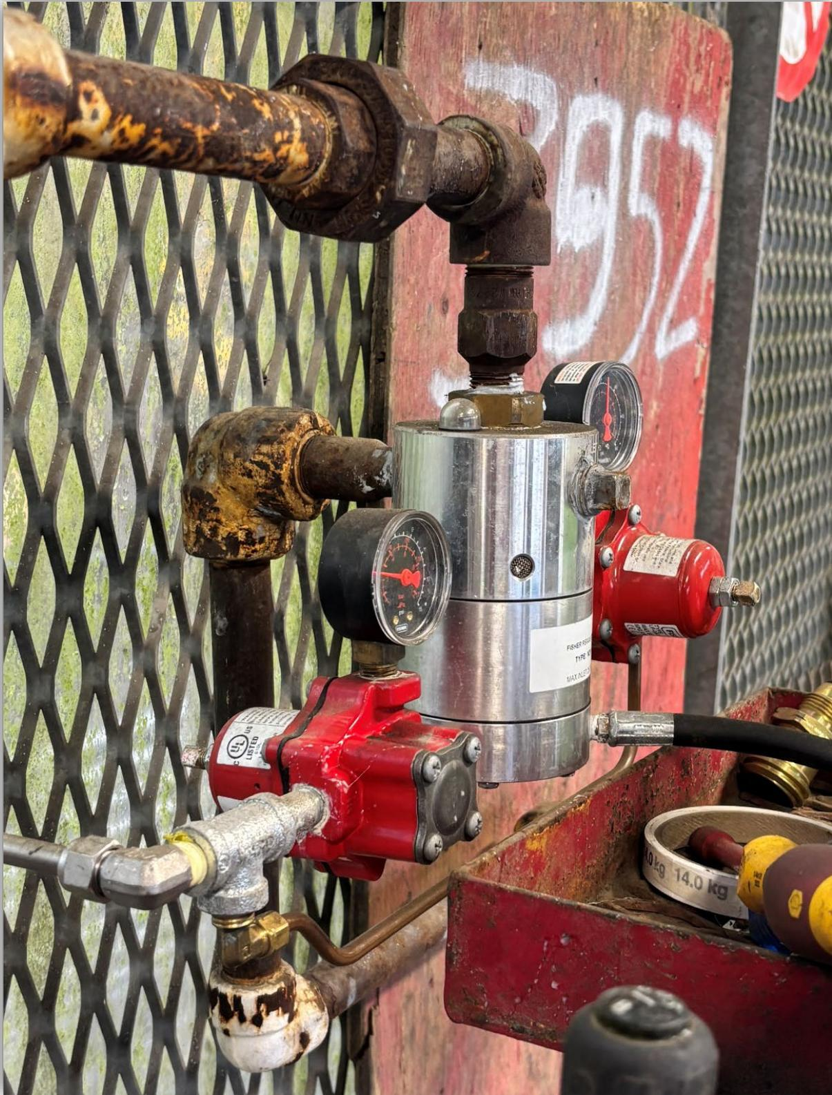
Image 10 – Fisher N201 automatic cylinder filling valve on one of the scales.
