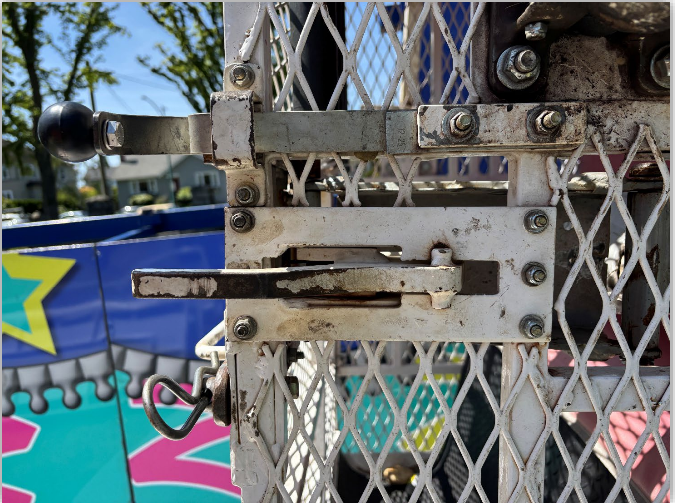
Image 3 – Door handle and latch on closed PCU door.
