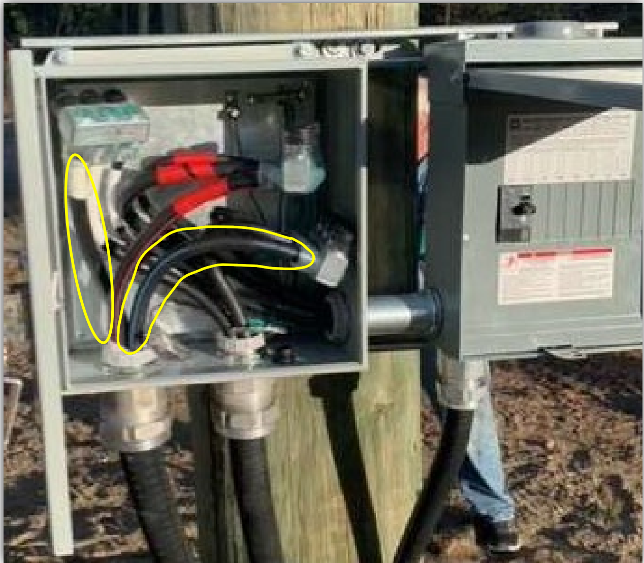
Image 2 - Junction box with splice to accommodate 100A panel on pole. [Circled] Misidentified conductors.
