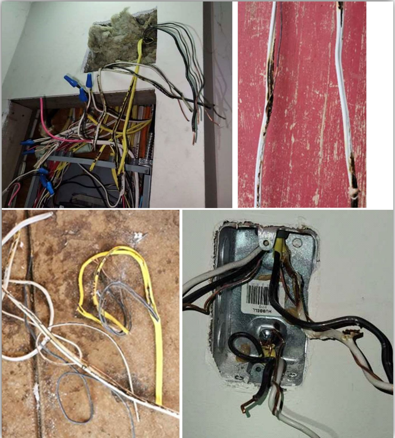
Image 3 - Damaged wiring inside the cabin.
