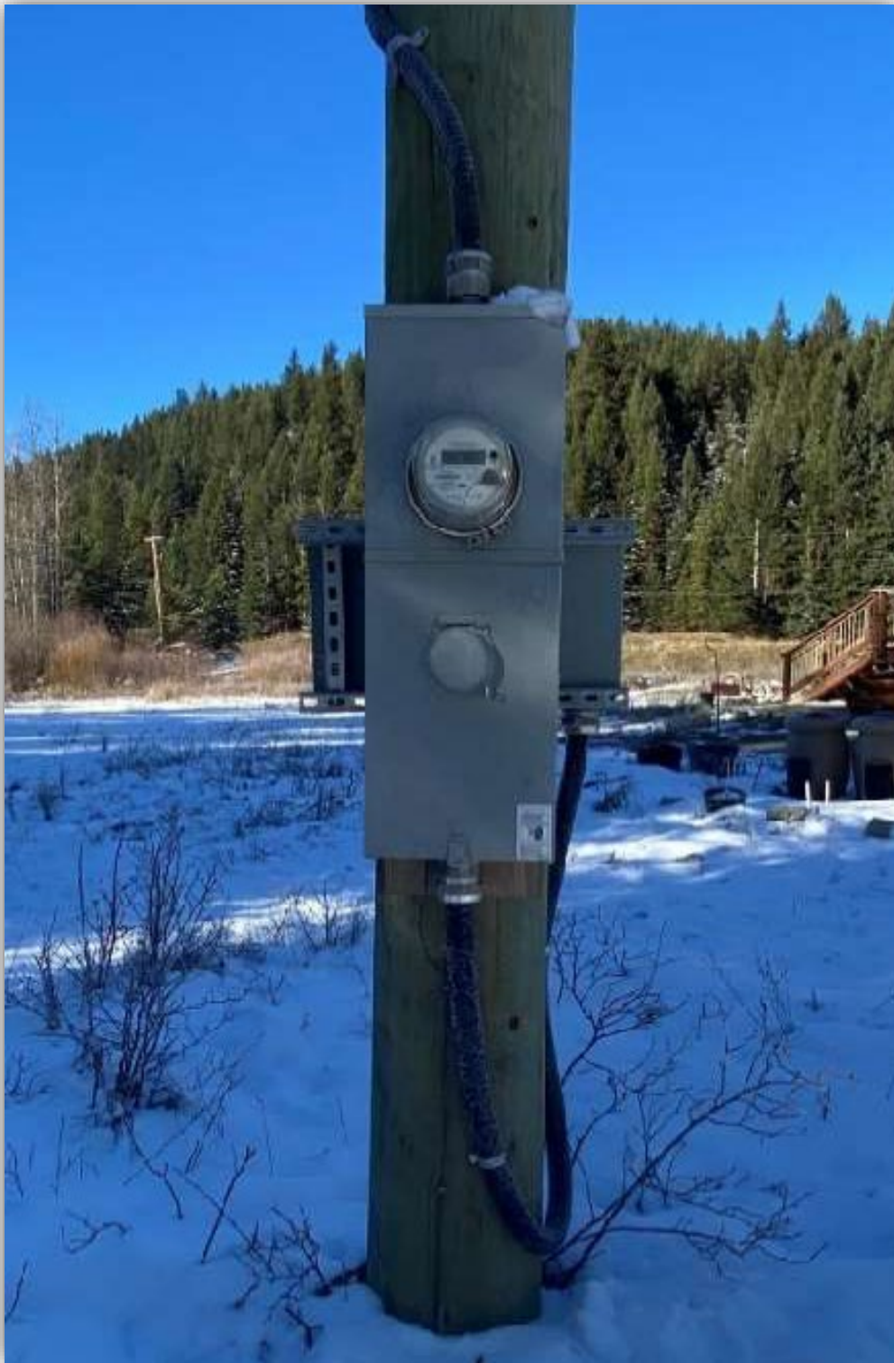
Image 1 - 200A combination meter with main breaker mounted to private pole.
