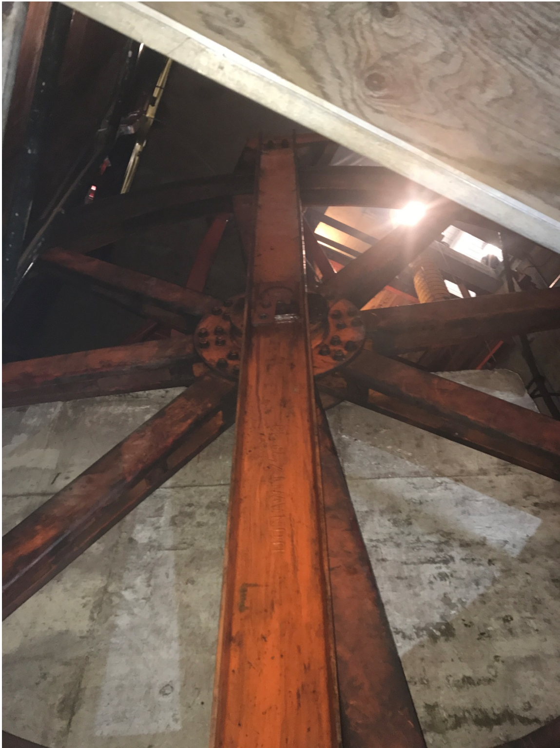
Figure 4, Photo of Bullwheel Configuration Prior to Upgrades
