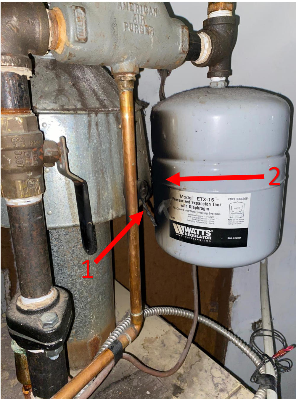
Image 5- Wires to the venting spill switch had been cut (1) and soot visible on expansion tank (2)
