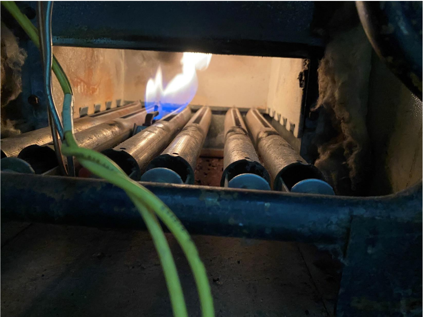
Image 7 – Boiler pilot flame in operation. The boiler operating manual states that a proper pilot flame is blue with the inner cone engulfing the thermocouple and an overfired pilot flame with lack of primary air will have a large lifting flame with a yellow flame tip as seen in the image and here: Pilot flame video .
