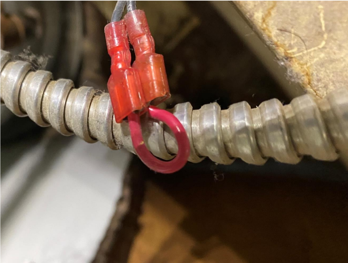
Image 2 – Jumper #1 electrical wire bypassing the draft hood spill switch
