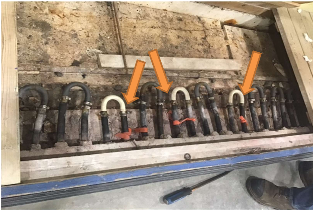
Image 11 Brine leaks off Brine Cycle at 1" 180° turns of ice sheet.
