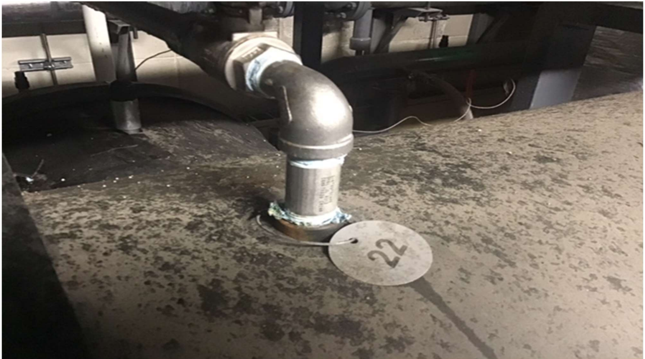
Image 4 Item number 22. Cool floor high point purge valve.
