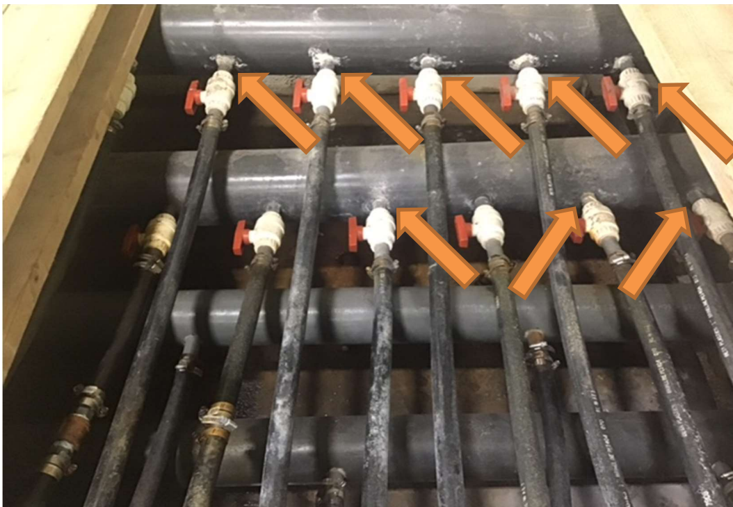
Image 12 Brine leaks off Brine Cycle at 1" outlets off 6" supply and return piping
