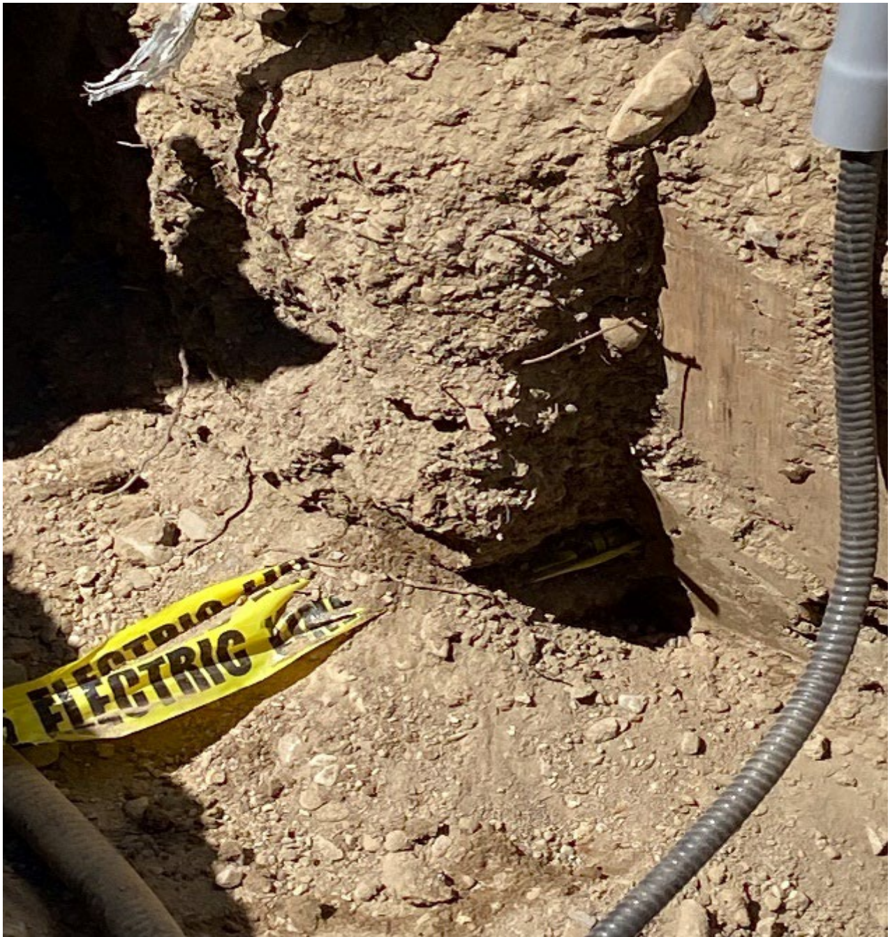
Photo 2 - Existing buried cable and burial tape coming away from building. Burial tape not installed at proper depth.
