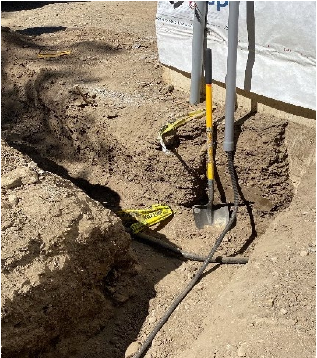
Photo 1 - Burial tape installed at time of original installation. Burial tape coming away from building and protruding from grade
