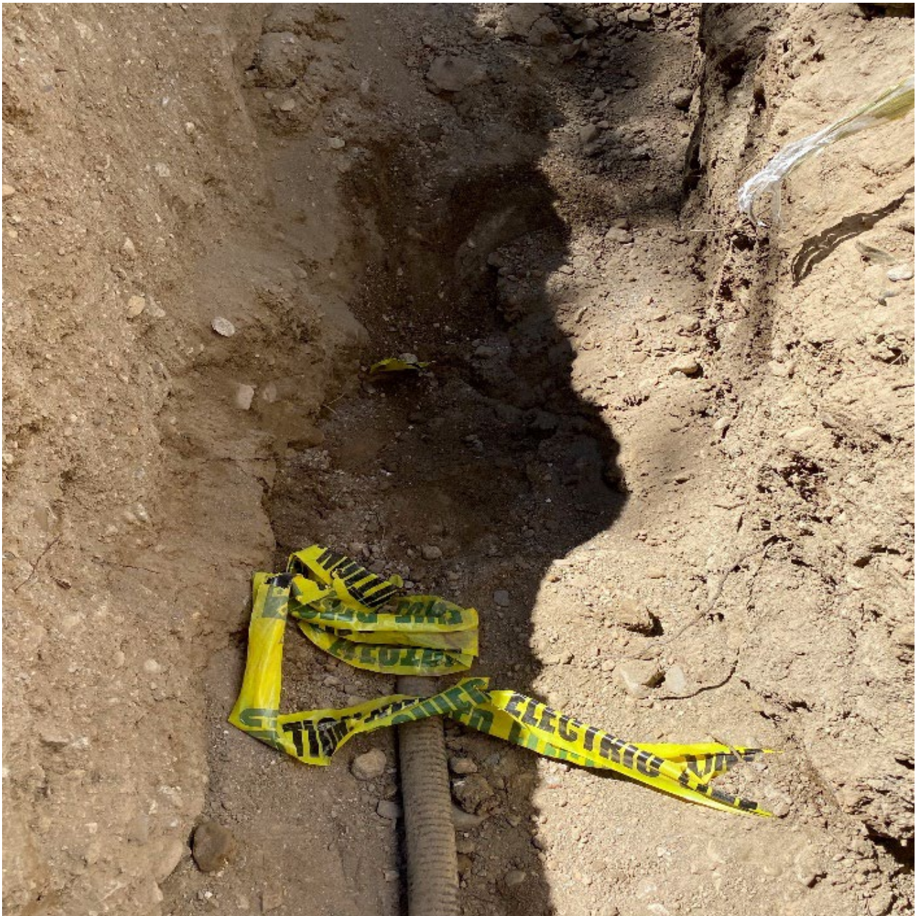
Photo 3 - Burial tape installed on top of sand and not half way between installation and grade.
