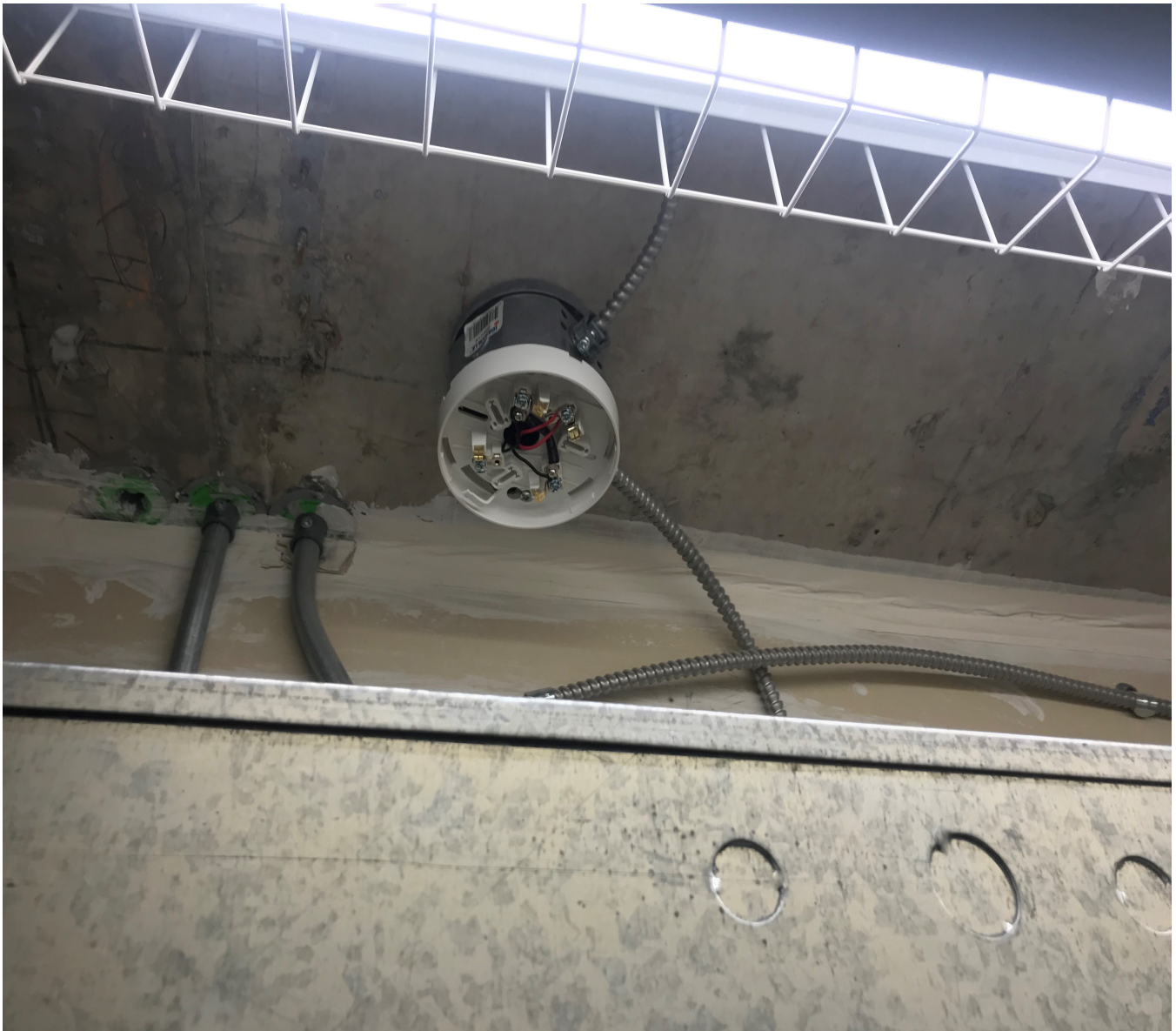
Photo 5: The smoke alarm located in the control space closet and installed directly above the affected resistor cabinet was melted during the incident. The damaged device was removed prior to site visit.
