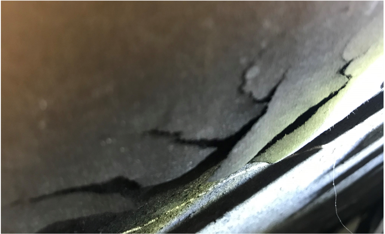
Photo 3: The top layer of drywall located behind the resistor cabinet that appears to have been scorched by radiant heat.
