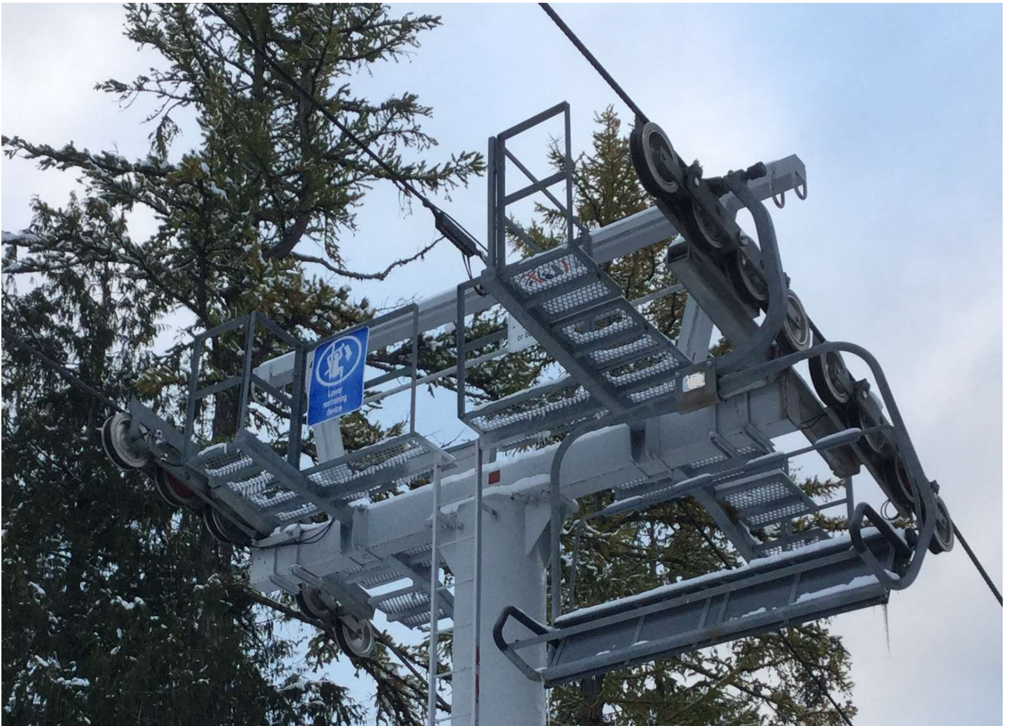
Figure 1, Tower and Sheave Assemblies
