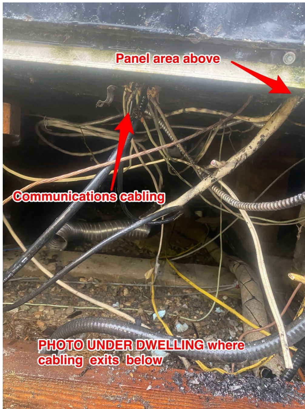
Image 3 – The crawlspace below the dwelling unit where cables are drawn into the finished wall space below the electrical panel. No evidence of fire noted in this area.
