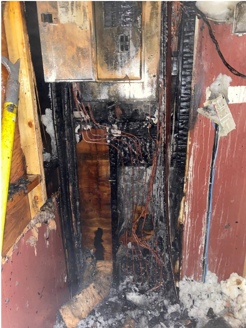
Image 6 - Shows wiring was installed to cross bracing near floor, limiting available wiring space for fished wires. Insulation is in place behind wires in wall, behind cross brace, higher up the wall, below the panel
