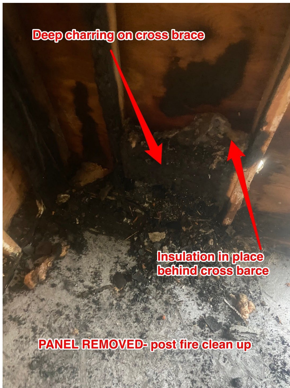
Image 5 - Lower section of wall - Area had original wiring and fished cabling run through this area with some in a tight space. A cross brace was in place leaving little depth for added cabling installed. Some insulation is noted behind lower cross brace
