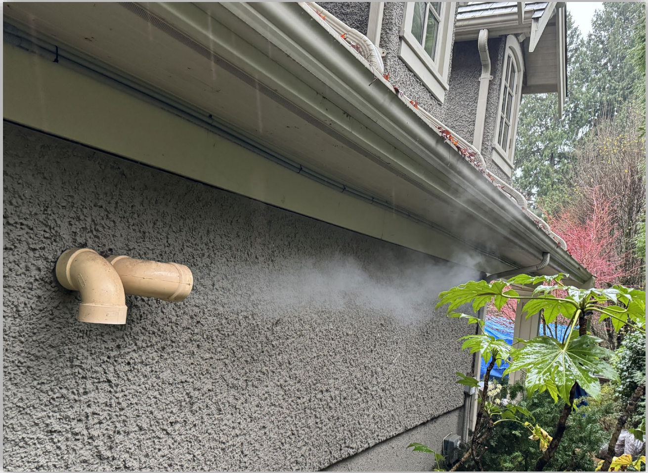
Image 4 - The boiler vent termination showing the flue gasses on high fire directed along side the house under the ventilated soffit.
