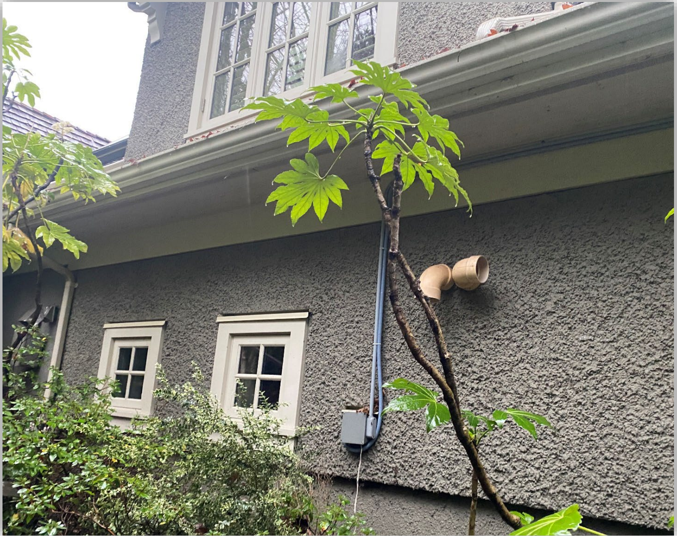
Image 3 - The boiler vent termination on the West side of the home.
