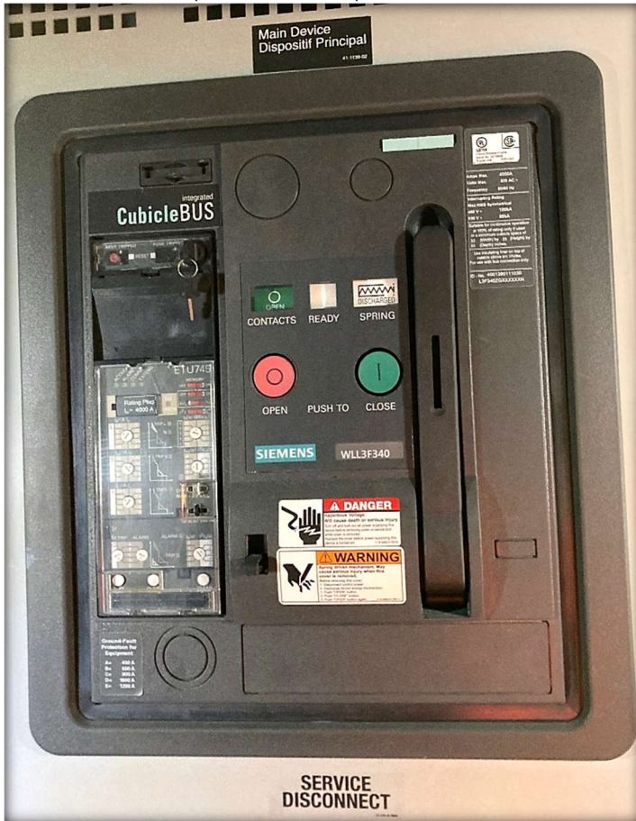
Figure 11 (top left) 600 Volt 4000 Amp MDC main breaker (Lockout location)
