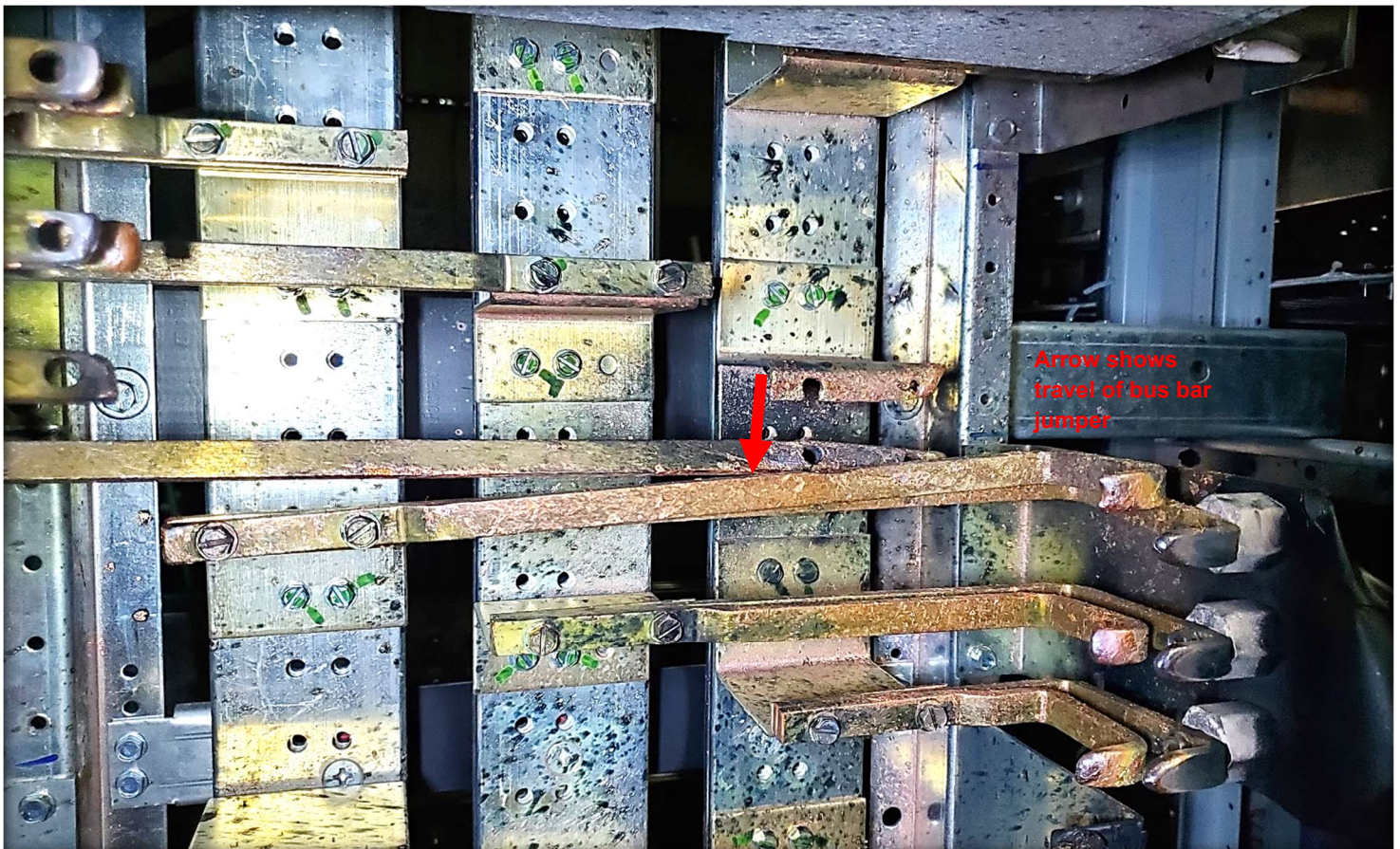
Figure 6 (bottom) – General area of arc flash showing damage to and travel of bus bar jumpers (arrow), and burn marks from arc flash
