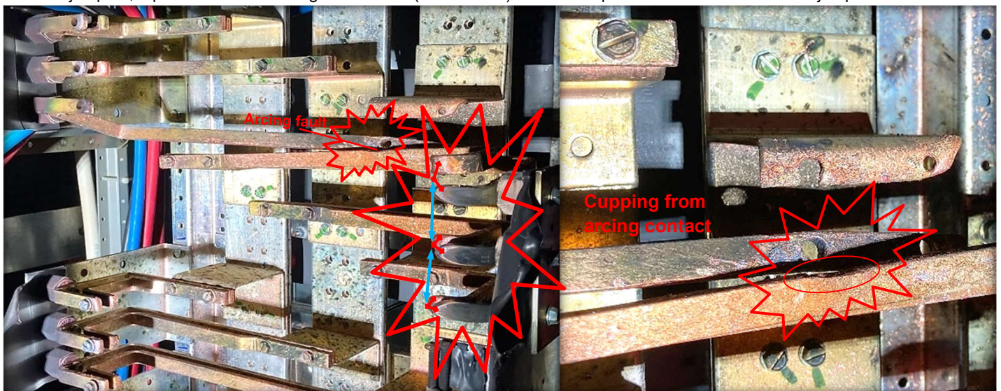
Figure 2 - (bottom left) Arc flash energy released at the ends of the bus bar jumpers, 3 phase arc flash through ionized air (blue arrows)
