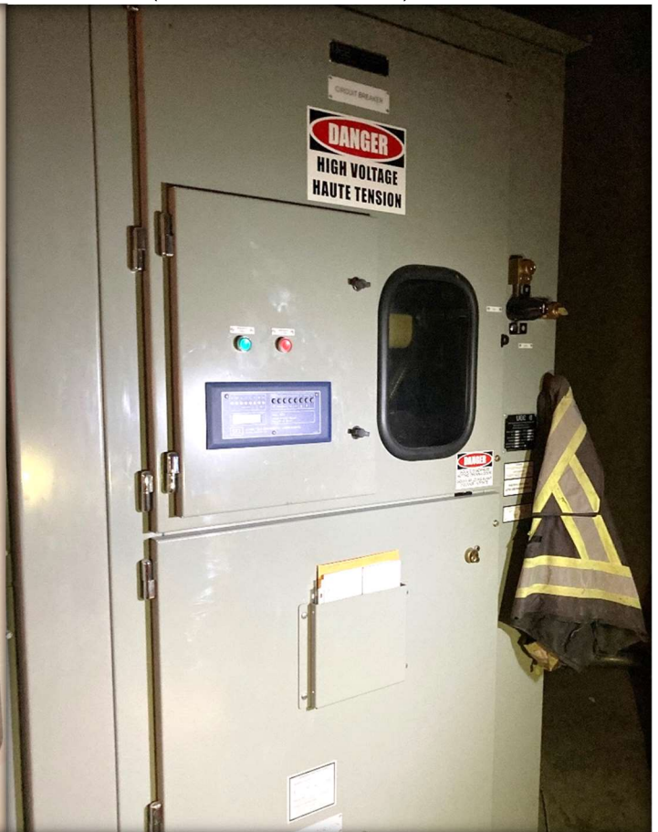
Figure 12 (top right) 25,000 Volt service switch (Alternate lockout location)
