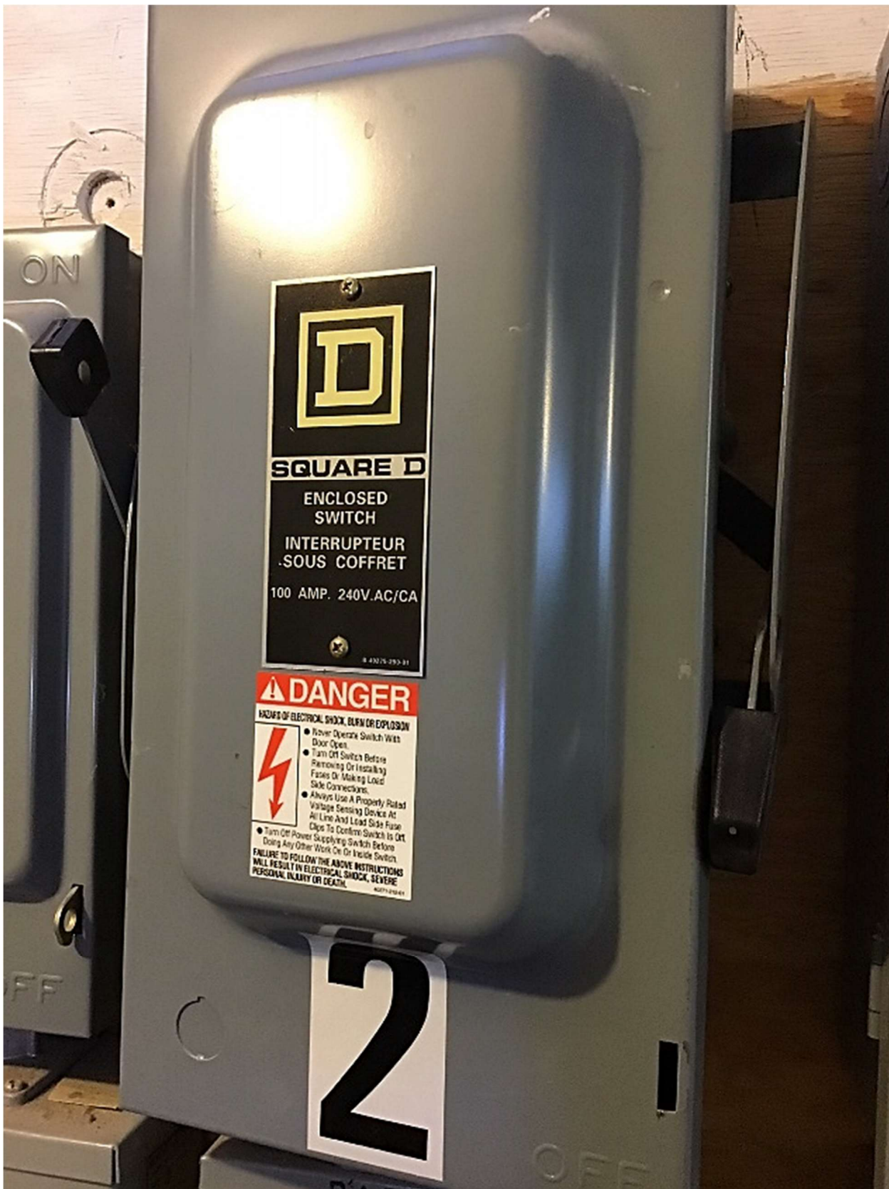
100A 240V fused disconnect supplying unit #2
