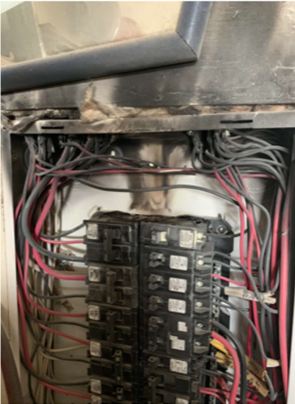
Image 1 - Burnt panel and wood above. The 30A 2-pole breaker is top left
