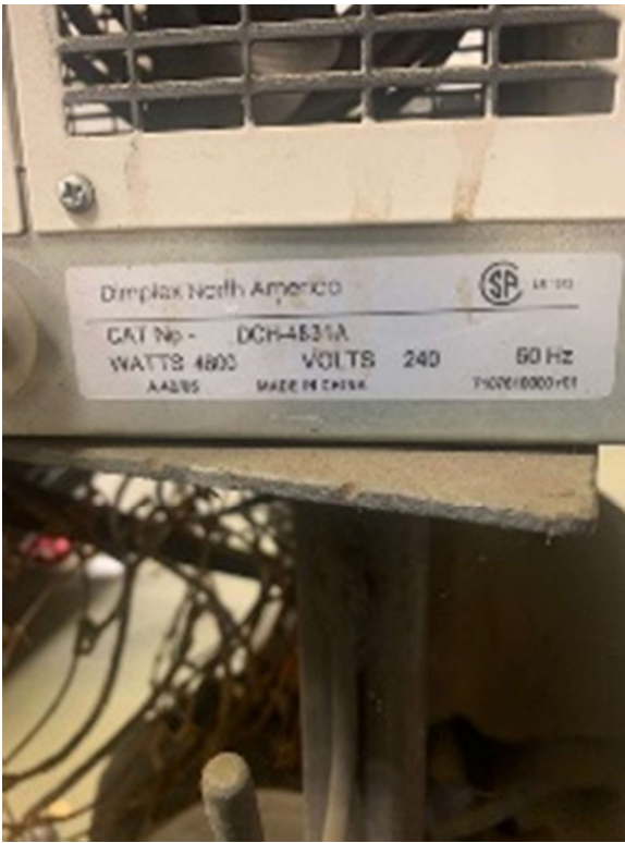
Image 3 - Construction Heater – 4800W
