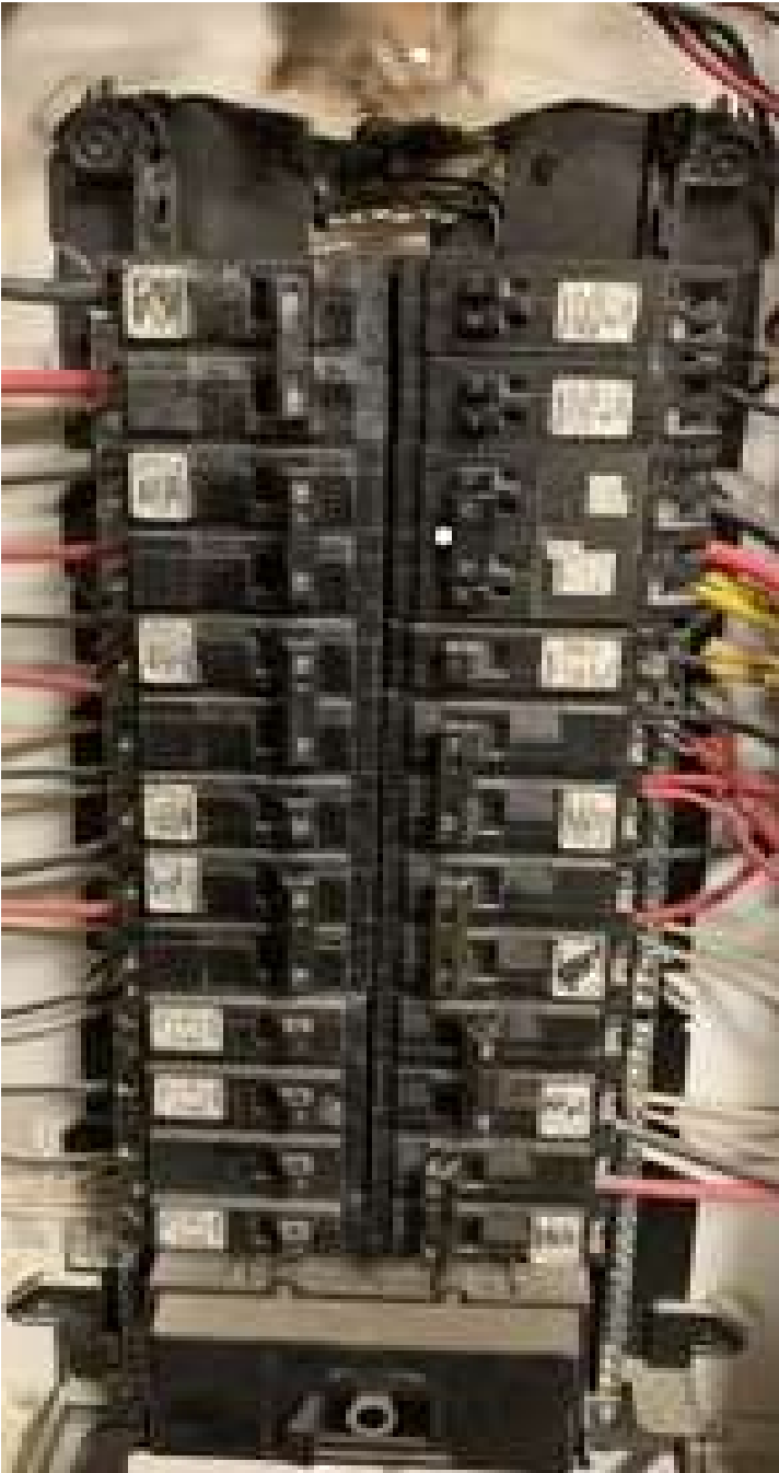
Image 2 - Burnt Panel with 30A breaker removed. Note melted buss top left.
