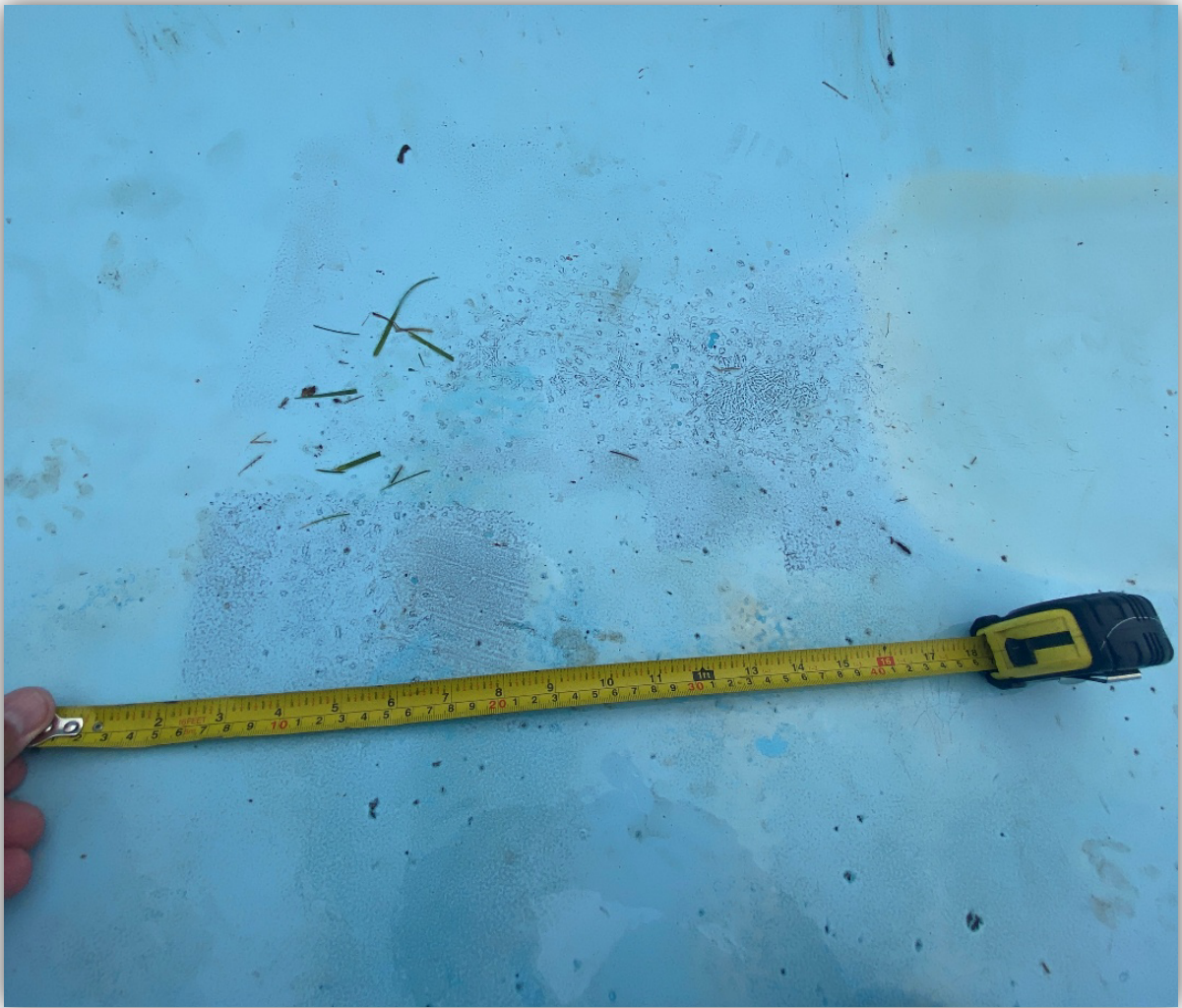
Image 9 – Exposed resin on one section of flume.
