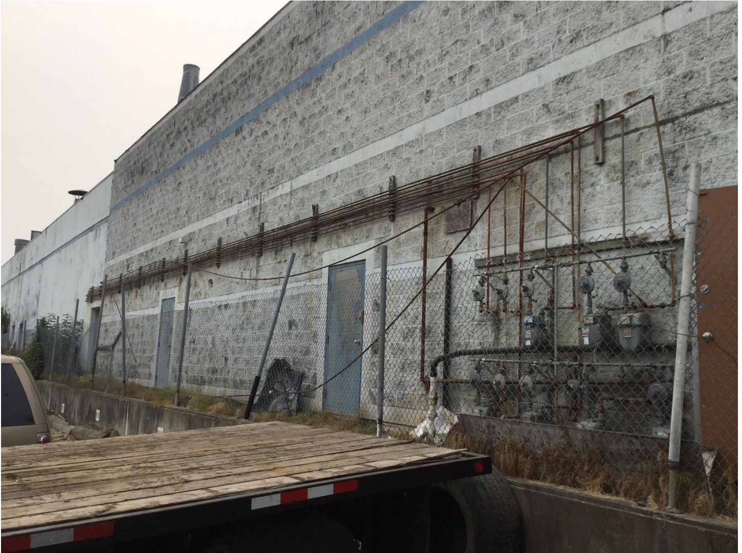
Fallen gas lines along side of Commercial building
