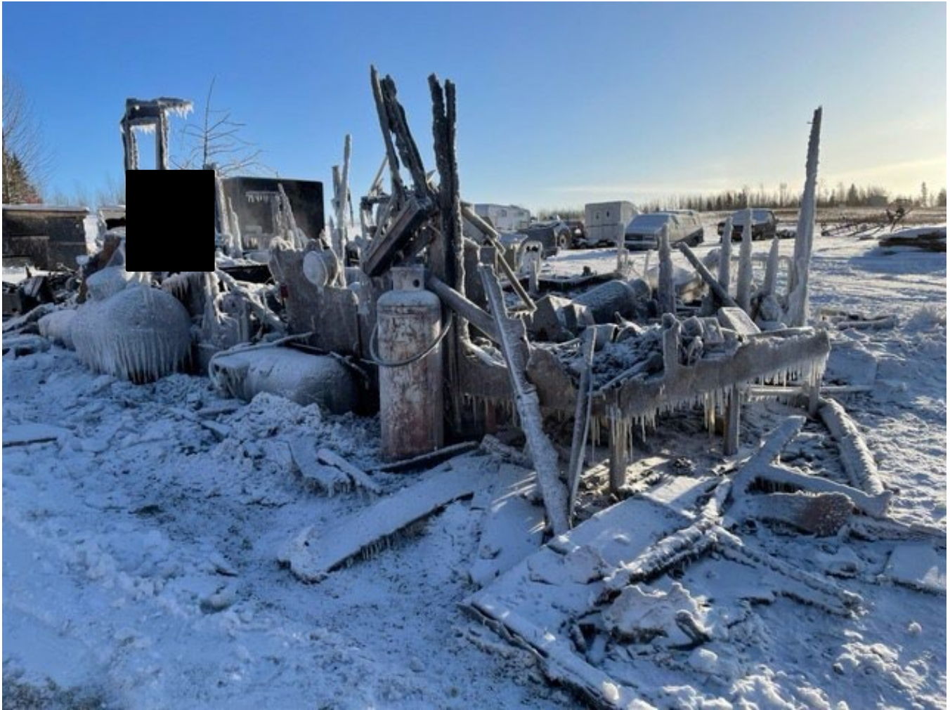
Photo 2 – The remaining structure of the residence showing multiple propane containers along the outside wall.
