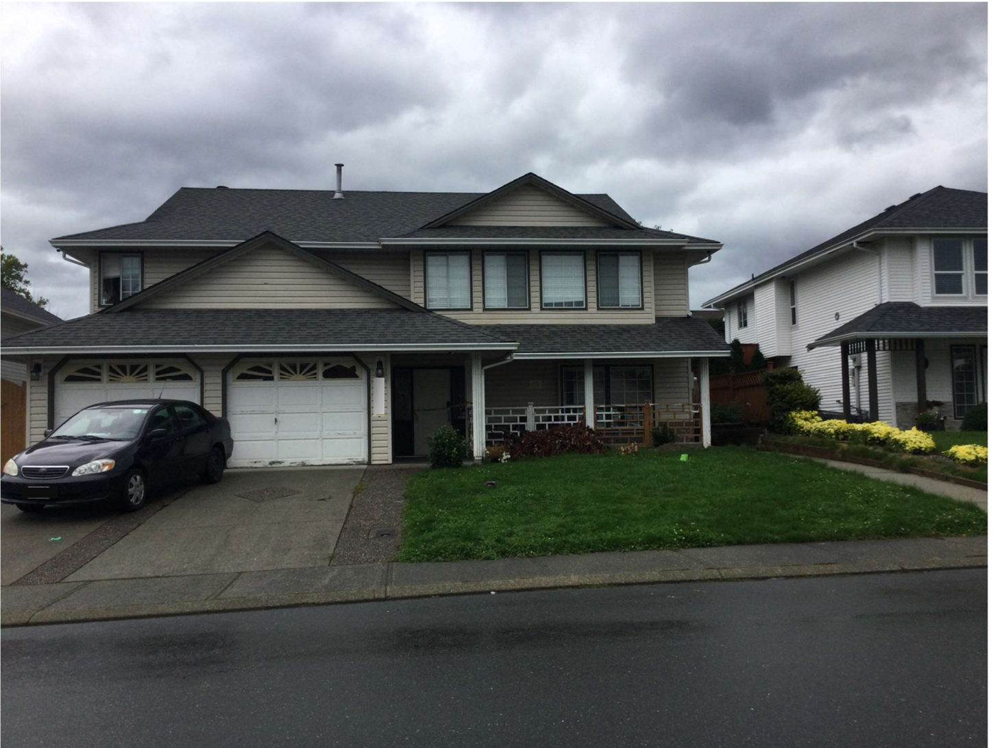
Picture 1- Front of the residential home.
