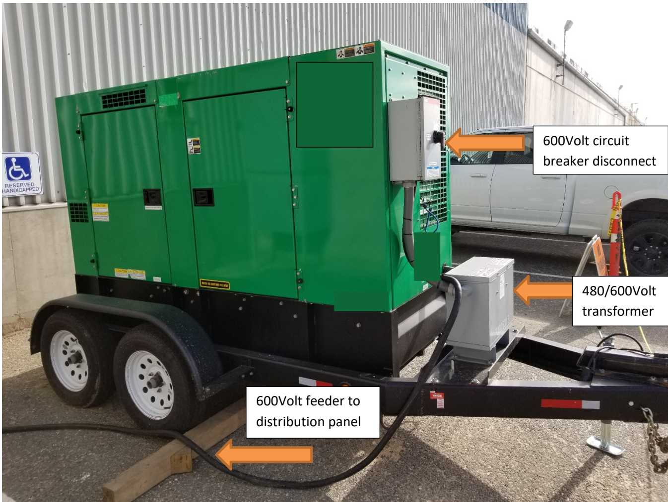
Image 1 - Generator set showing 480/600-Volt transformer and disconnect.
