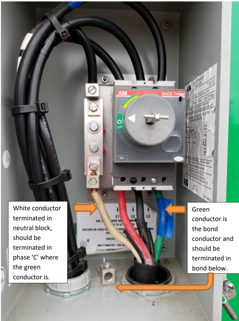
Image 3 - Incorrect wiring of cable in 600-Volt circuit breaker disconnect.
