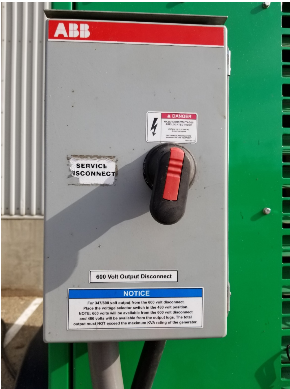
Image 2 - 600Volt circuit breaker disconnect.
