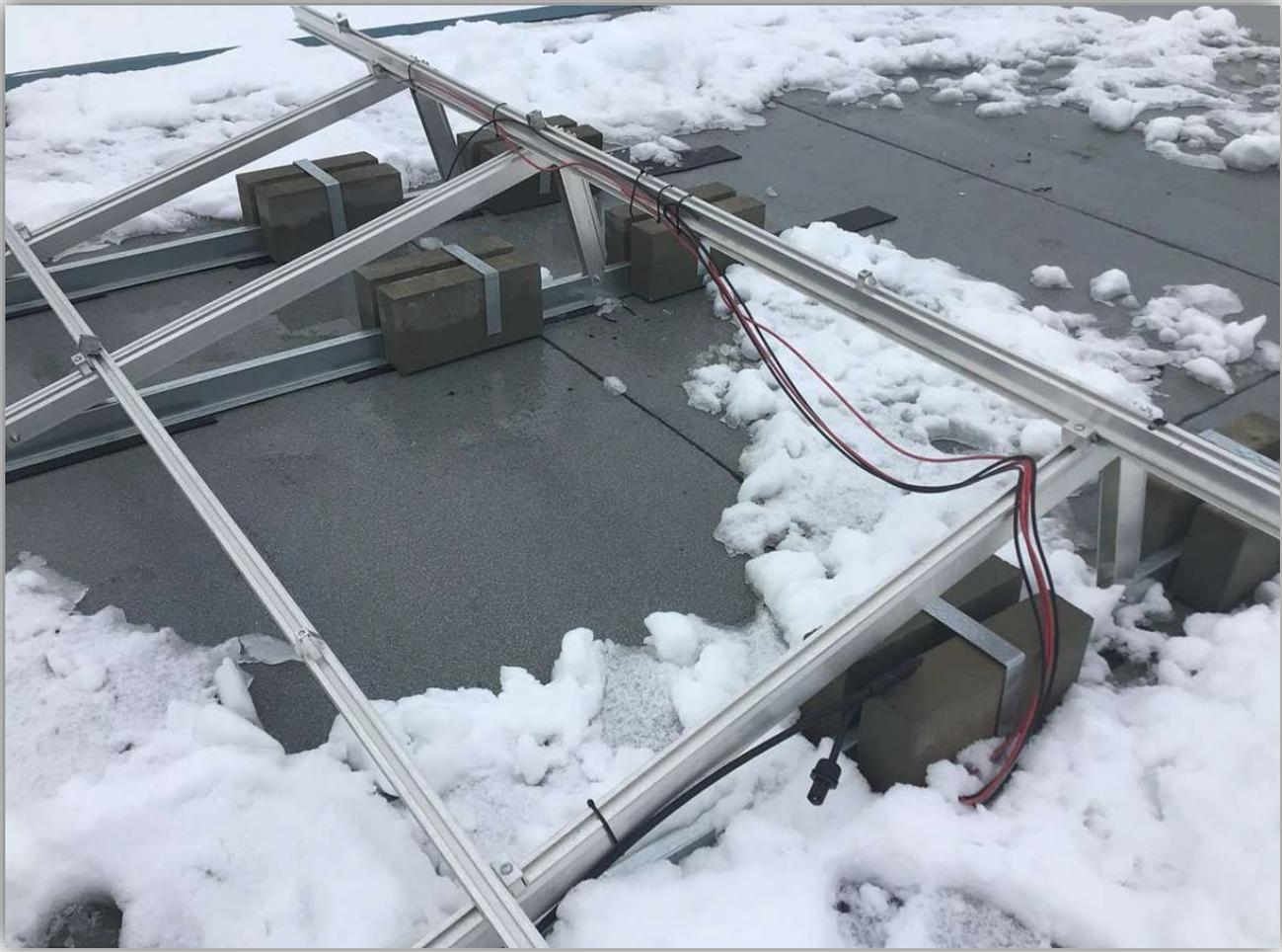
Image 2 - Weighted ballast installation methods for this array. Two ballasts float over a metal channel plate and are secured together by a metal strap.
