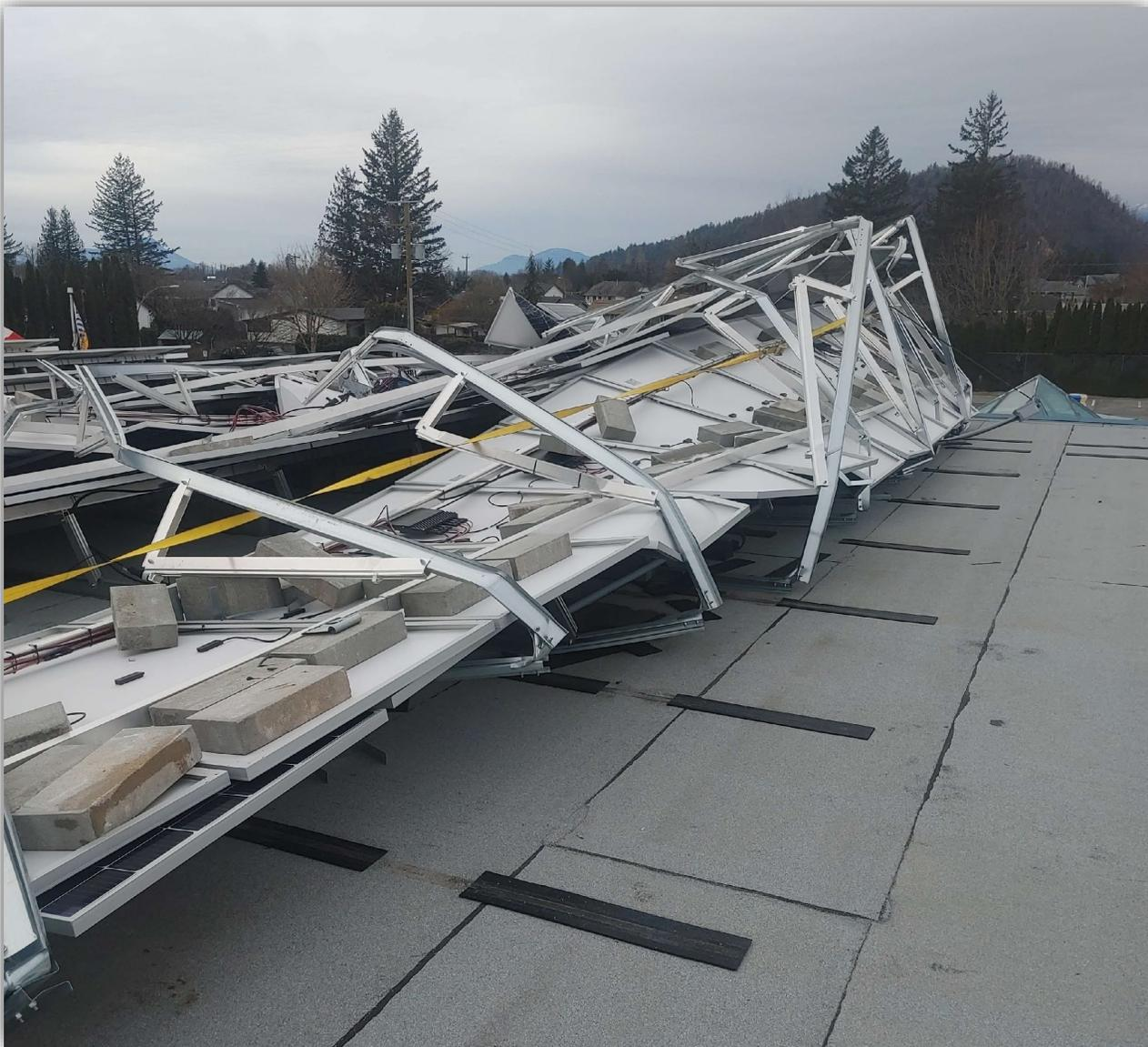
Image 1 - Effects of windstorm overcoming the weight of the concrete weighted ballasts and uplifting the solar array (concrete ballasts visible).
